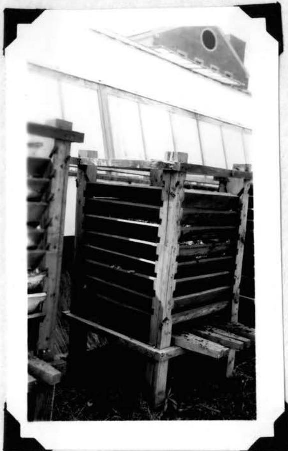
Figure 2. An Activated Compost Frame With The Solid Sides Removed to Show Details of Construction.
