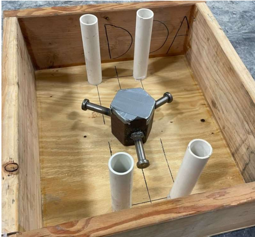
Figure 39 - Support B before being casted.
