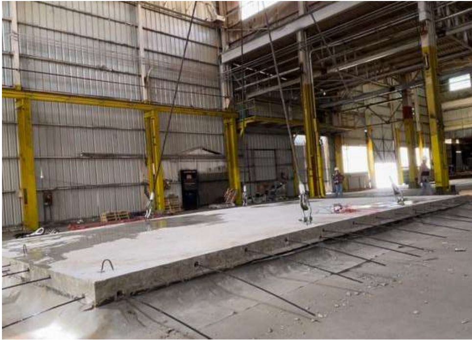
Figure 72 - Full-scale slab being picked up by the four middle hooks.
