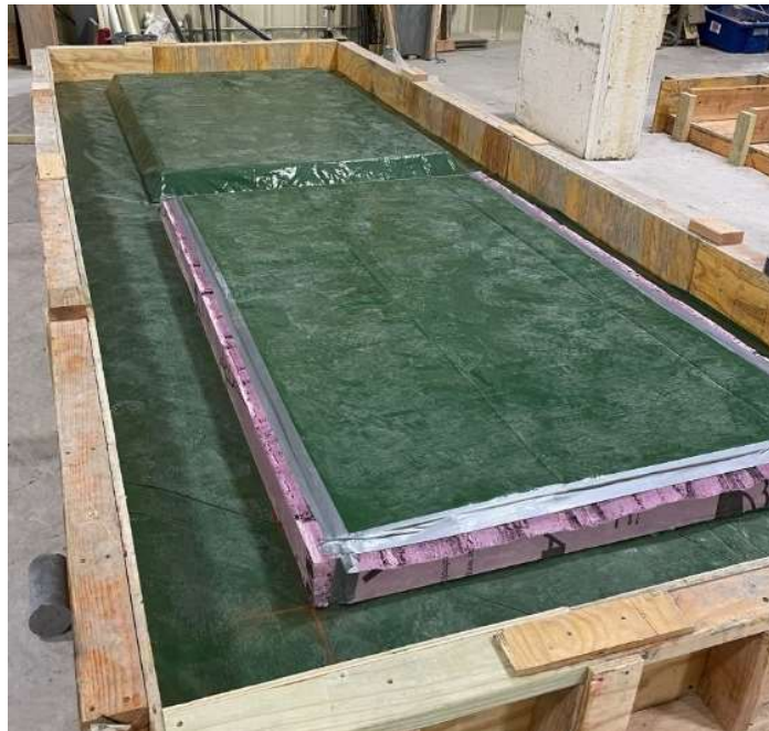
Figure 26 - Formwork for scaled prototype showing both types of inserts.
