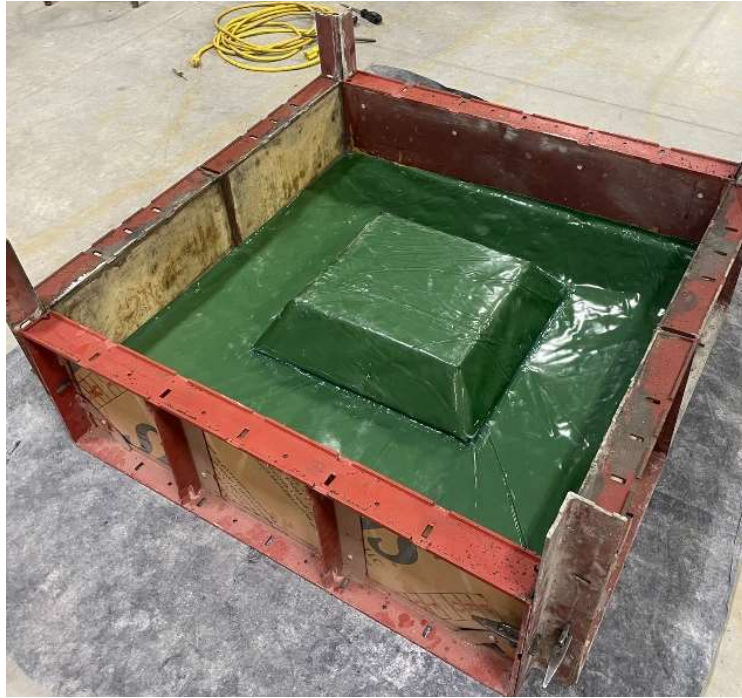
Figure 25 - Second insert formwork prototype.
