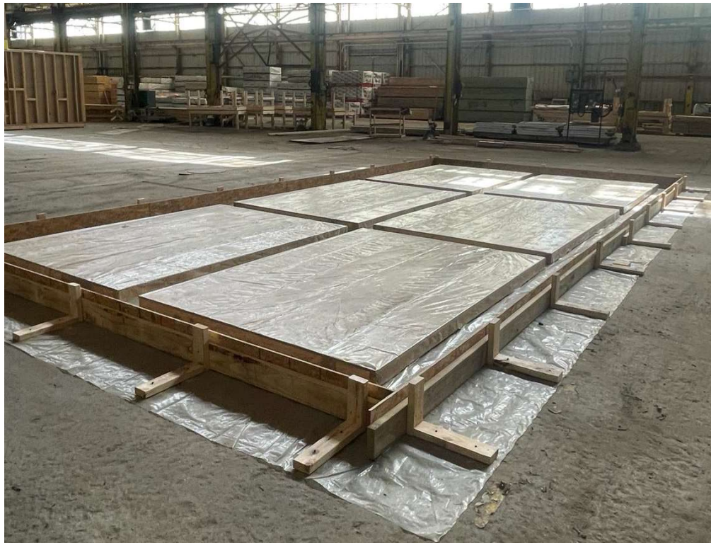
Figure 40 - Formwork of full-scale slab.
