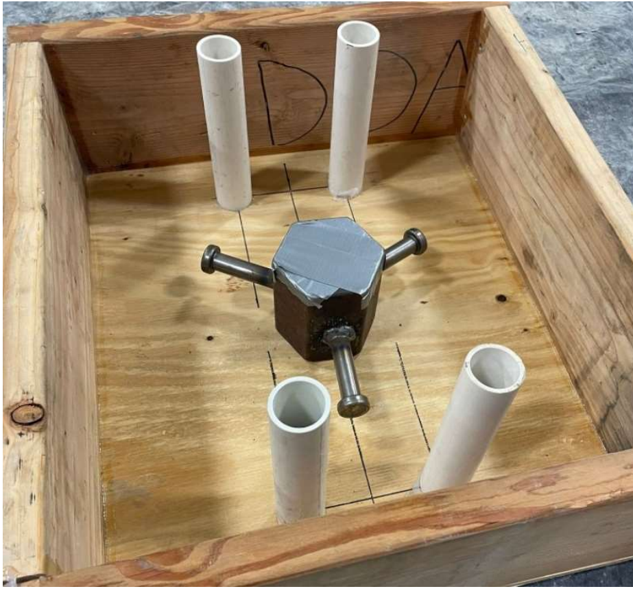
Figure 78 - Support option B inside formwork before concrete was cast.
