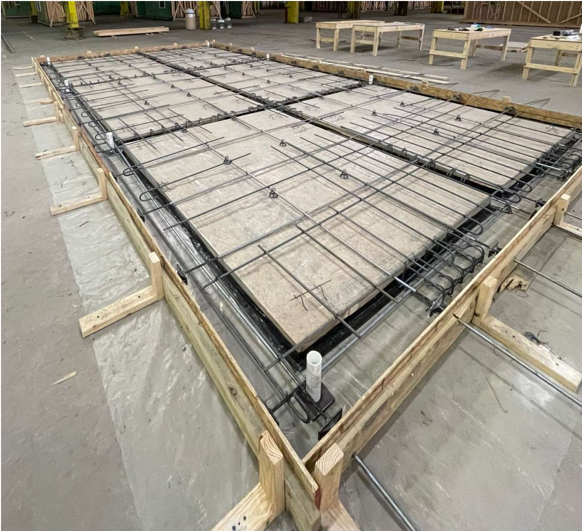
Figure 41 - Formwork, reinforcement, tendons, and sleeves in place for full-scale prototype's casting.
