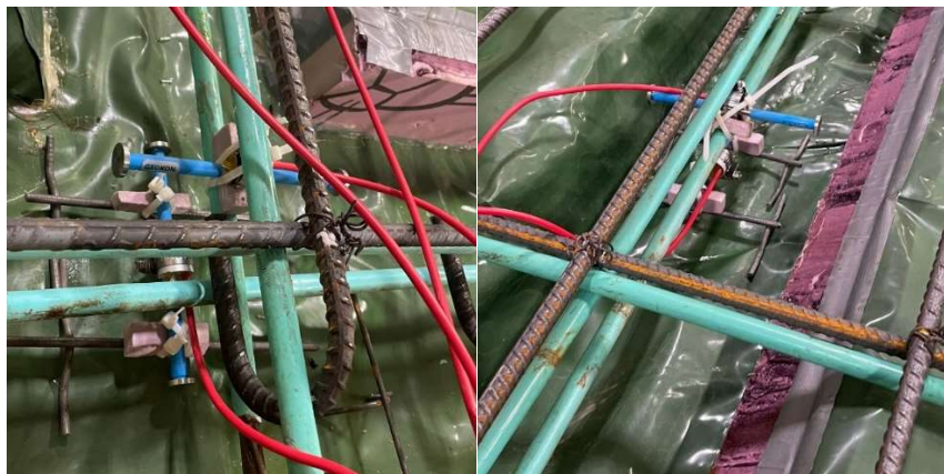
Figure 31 - Installation of VWSGs in scaled prototype.
