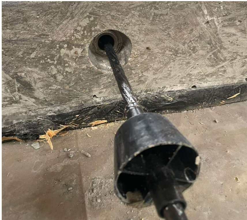
Figure 28 - Space left by pocket formers once removed from the slab.
