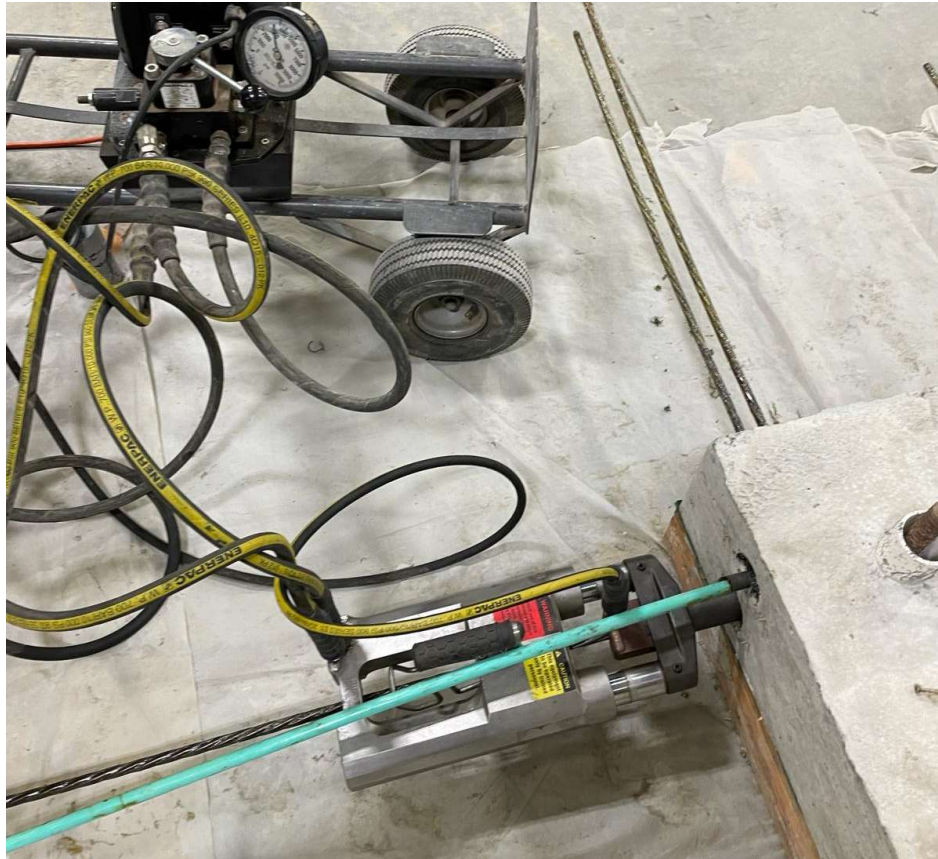
Figure 35 - Post-tensioning of tendons using hydraulic jack on scaled prototype.
