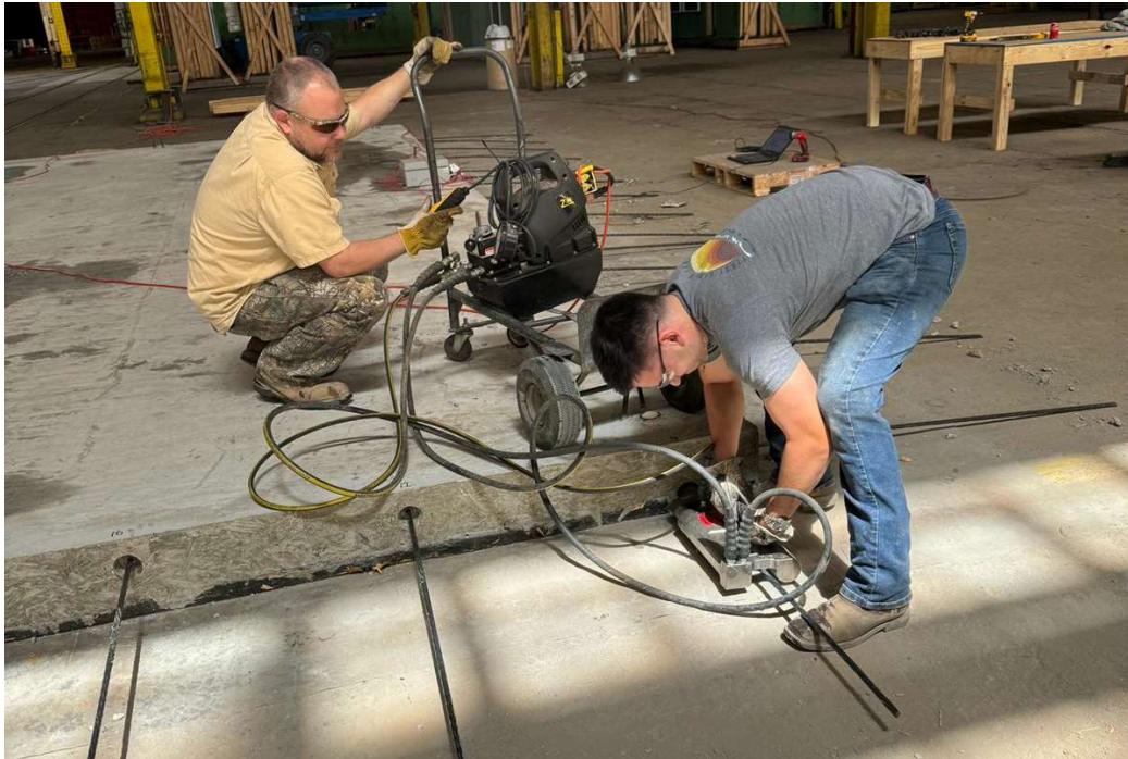
Figure 46 - Post-tensioning of tendons using hydraulic jack on full-scale prototype.
