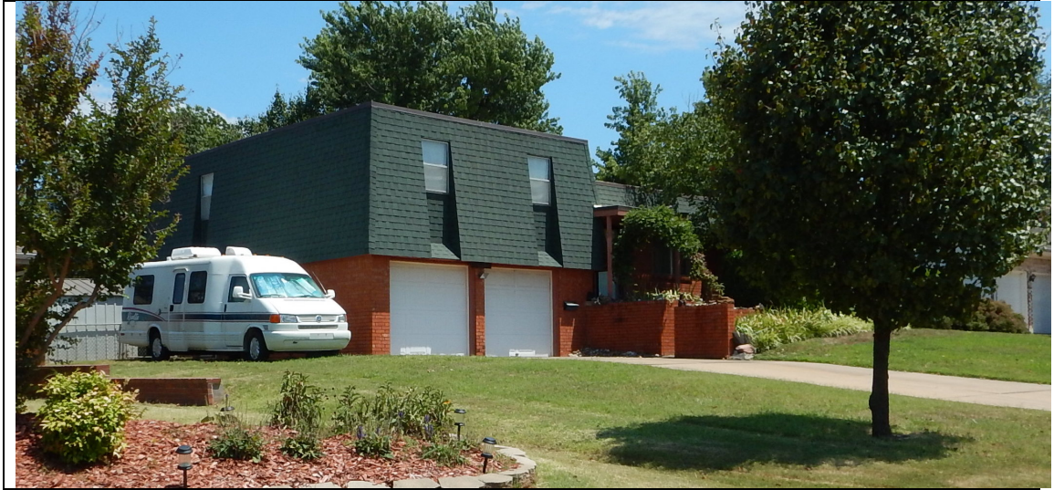
#063 701 NORTH MANNING STREET (b. 1972) Warrants Further Study (Criterion C, Local Significance)
