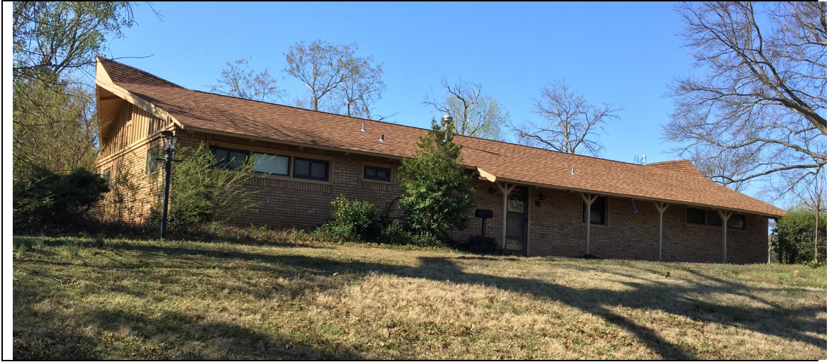
#032 913 WEST LAKERIDGE AVENUE (b. 1956) Warrants Further Study (Criterion C, Local Significance)
