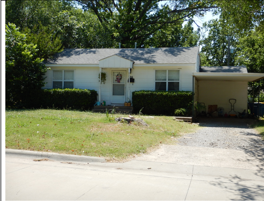
Figure 8. Typical Minimal Traditional Cottage. The Erma Payne Fowler Home, built in 1948, located at 206 South Arrington in the Highland Park area, contains 1,080 feet and has three bedrooms.
