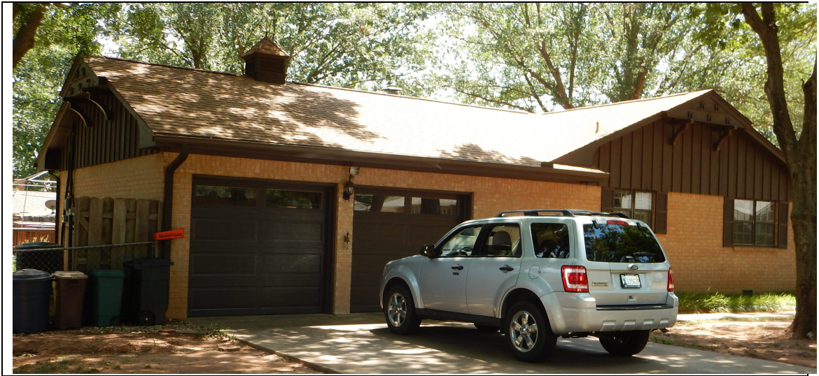
#062 301 NORTH MANNING STREET (b. 1968) Warrants Further Study (Criterion C, Local Significance)
