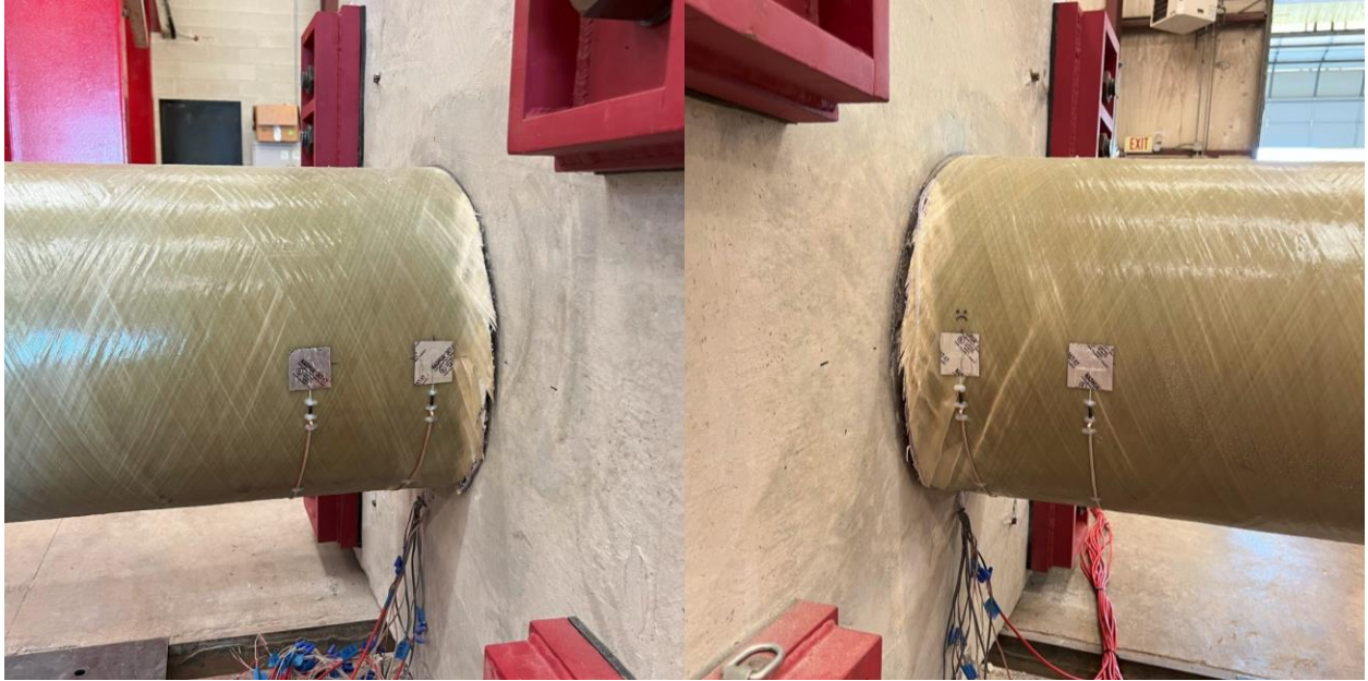
Figure 5-23: HS-SCC 2 GFRP Tube West Side (l) and East Side (r) Damage After Testing
