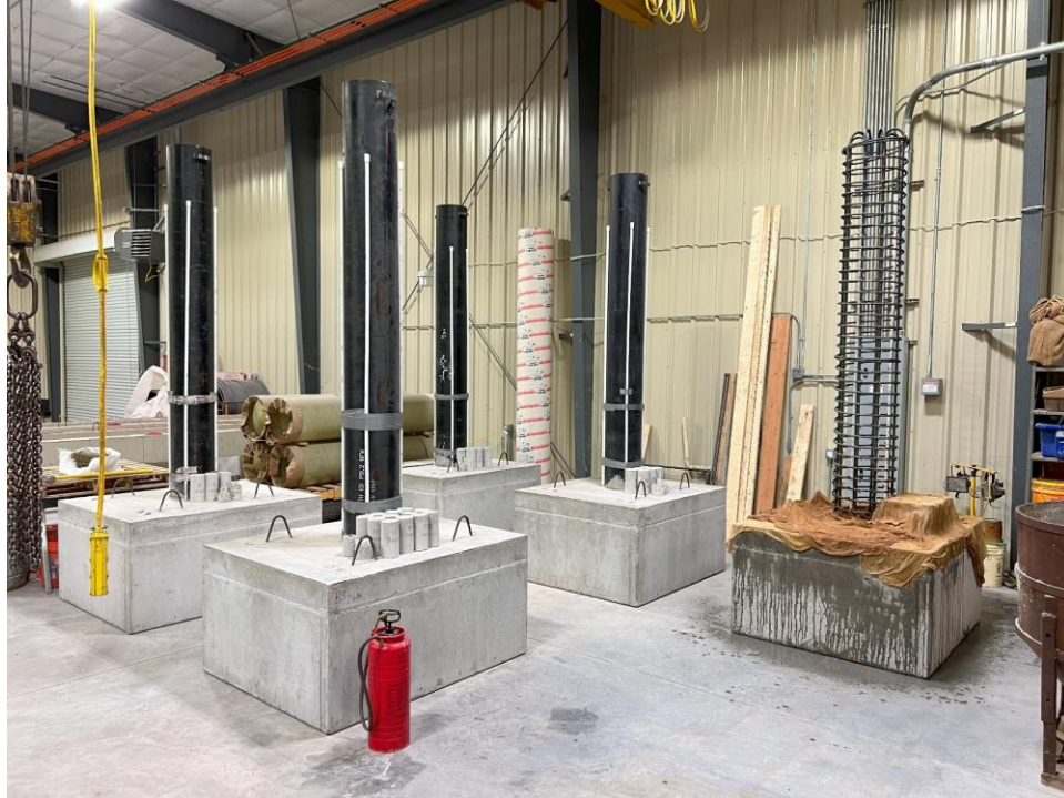
Figure 4-20: Completed Column Bases
