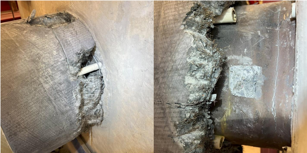
Figure 7-13: UHPC 1 Concrete Core After Light (l) and Significant (r) Concrete Removal
