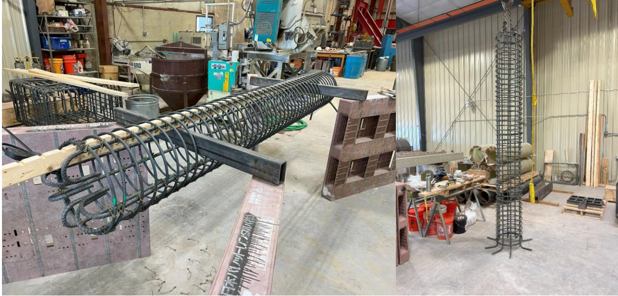
Figure 4-3: Assembled Spiral-Tied Reinforcement Cage, Horizontal Construction (l) and Titled Upright (r)
