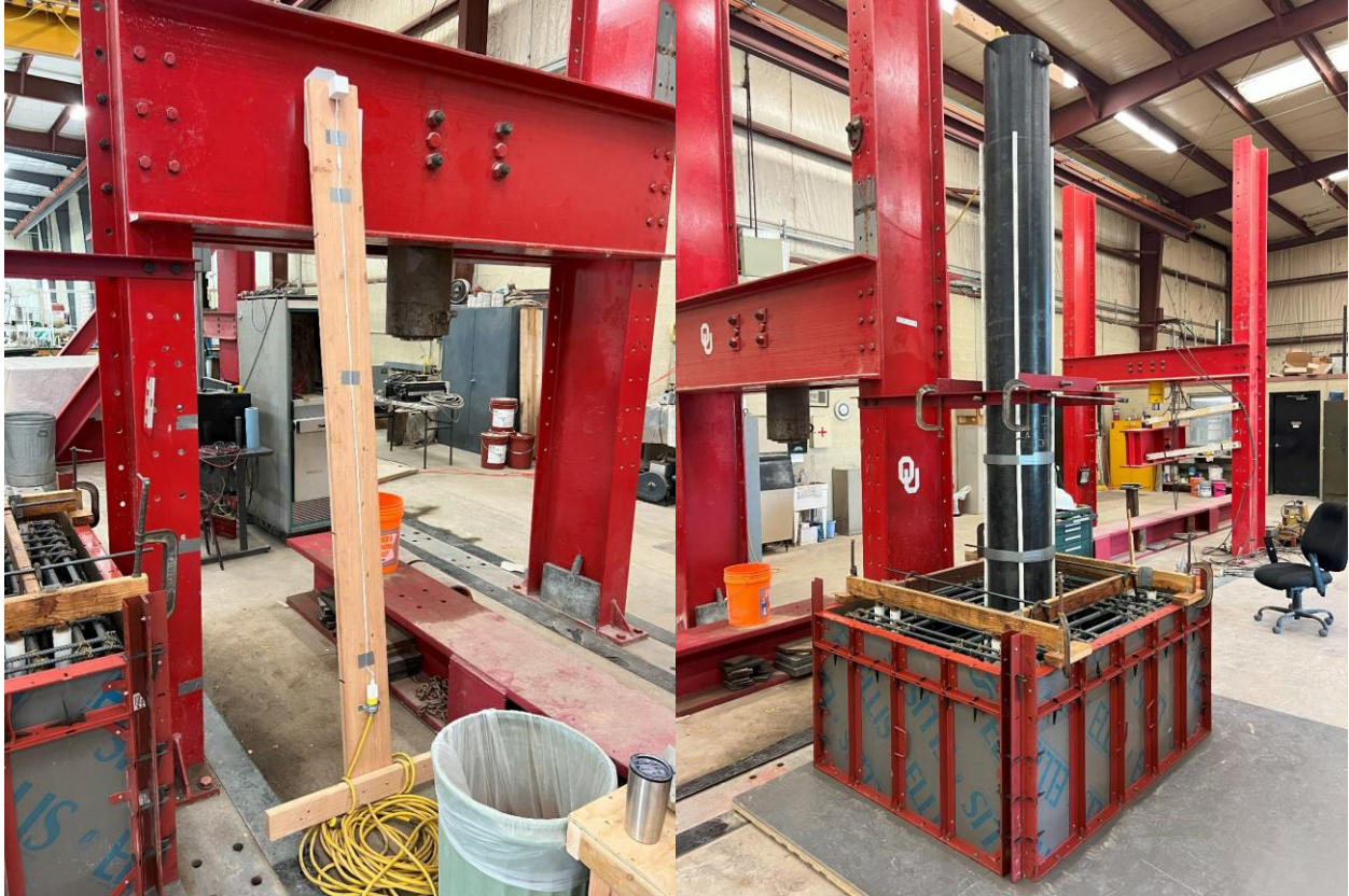
Figure 4-15: HC-FCS Base Assembly, Camera for Monitoring Internal Concrete Level (l) and Finalized Specimen Ready for Casting (r)
