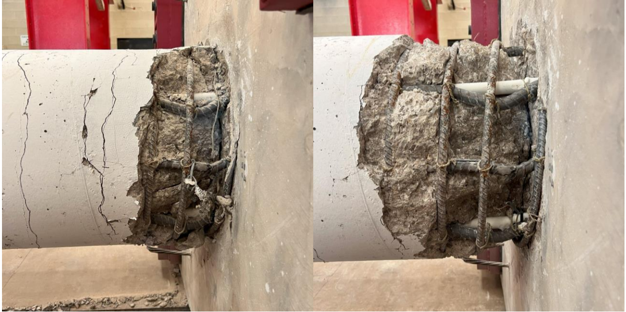
Figure 5-7: RC Column West Side After Testing (l) and Removal of Loose Concrete (r)
