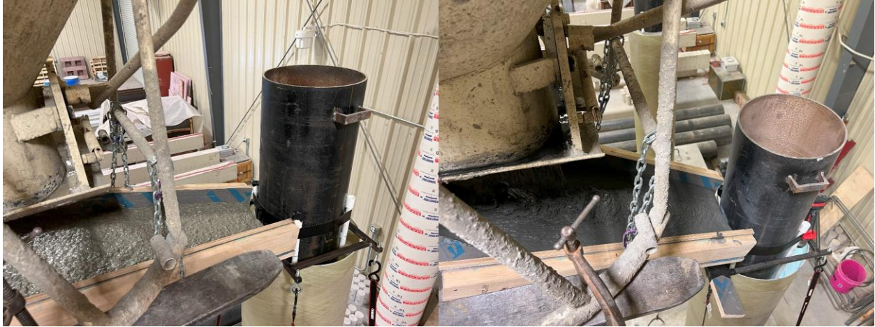
Figure 4-29: HC-FCS Column Casting, HS-SCC Core (l) and UHPC Core (r)
