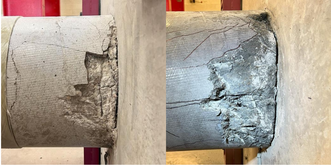
Figure 8-12: Comparing HS-SCC 2 (l) and UHPC 2 (r) Concrete Core West Side After Testing and Light Removal of Concrete
