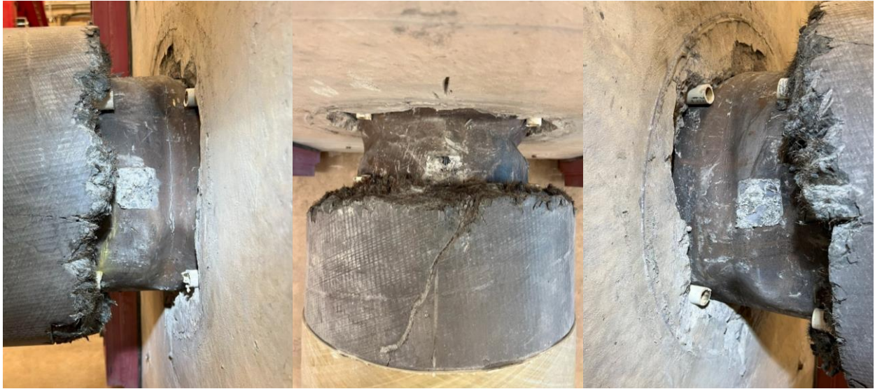
Figure 5-34: UHPC 1 Steel Tube West (l), Top (m), and East Side (r) Damage After Testing
