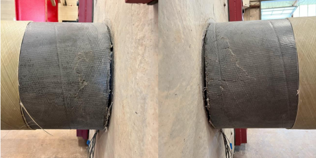
Figure 5-33: UHPC 1 Concrete Core West Side (l) and East Side (r) Damage After Testing
