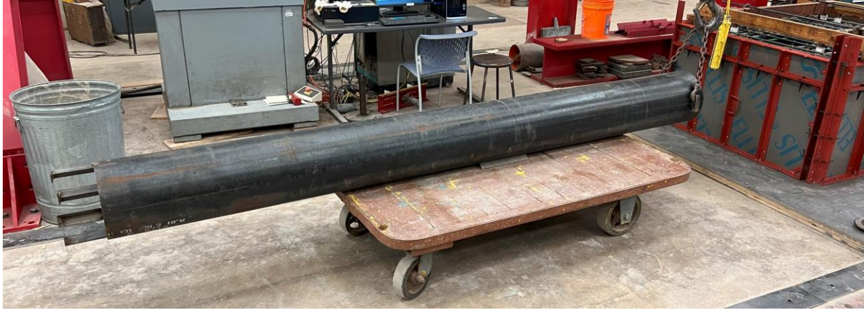
Figure 4-7: Completed Steel Tube Ready to be Tilted and Placed
