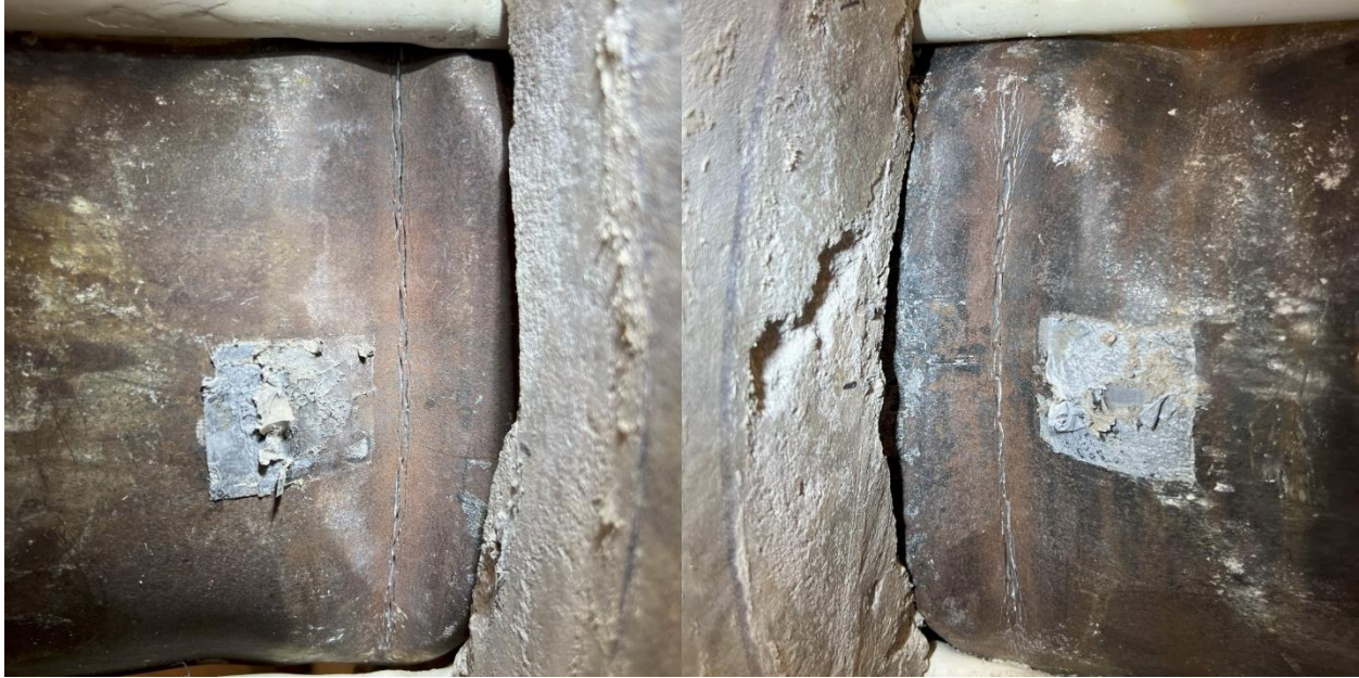
Figure 6-27: HS-SCC 2 Steel Tube West (l) and East Side (r) Damage After Testing
