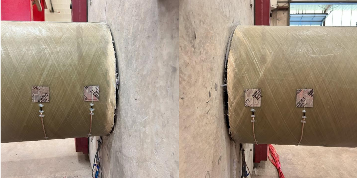
Figure 7-24: UHPC 2 GFRP Tube West Side (l) and East Side (r) Damage After Testing
