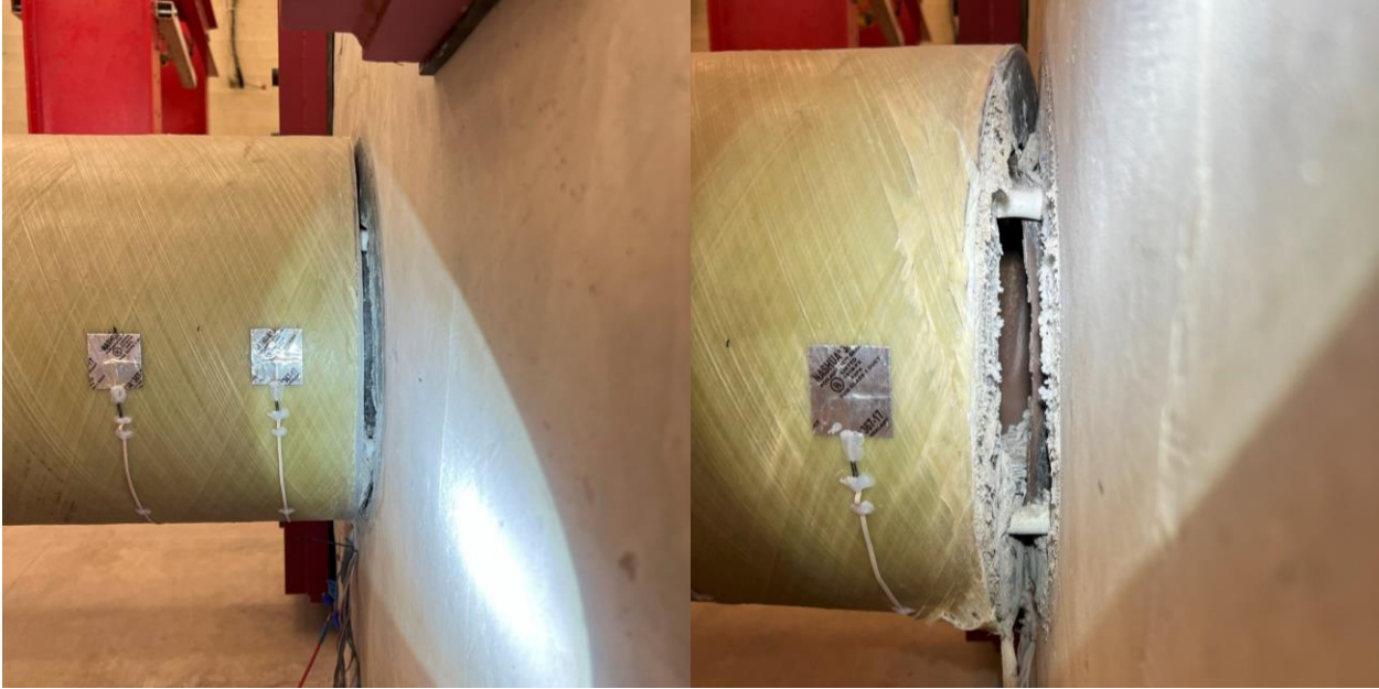
Figure 5-14: HS-SCC 1 Column Separation and Fractured Steel Tube During Testing
