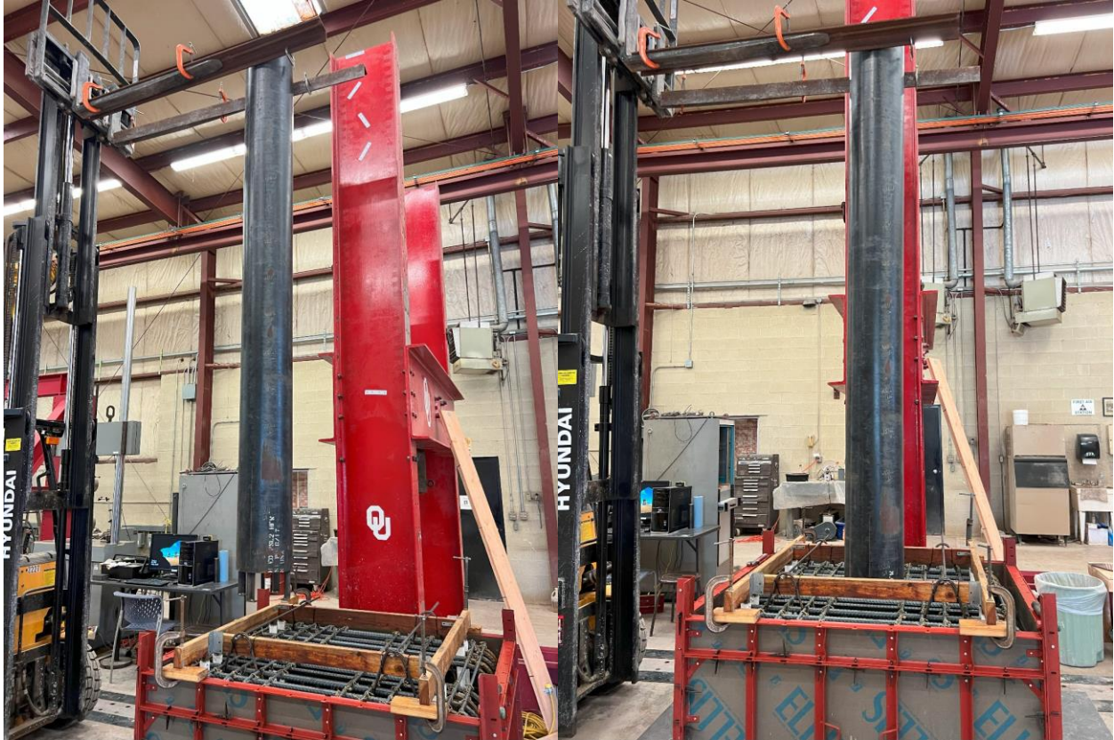
Figure 4-14: Steel Tube Placement, Lifting with the Forklift (l) and Insertion into the Reinforcement Cage (r)
