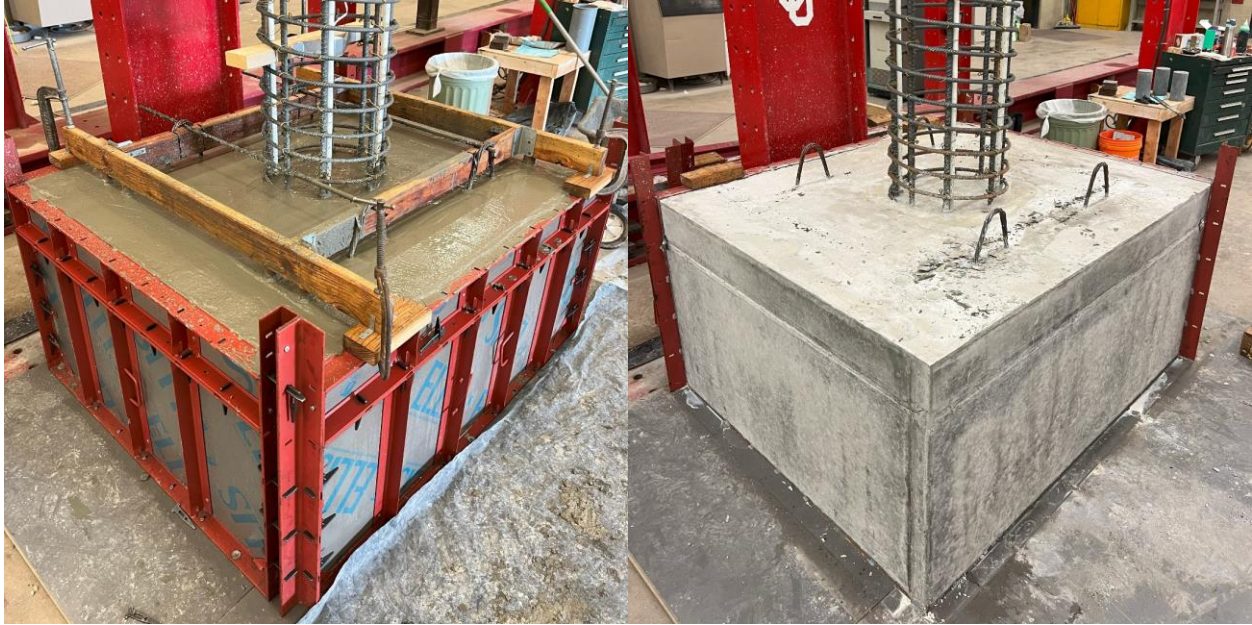
Figure 4-18: RC Column Base Construction, Immediately After Casting and Finishing (l) and After Stripping the Formwork (r)
