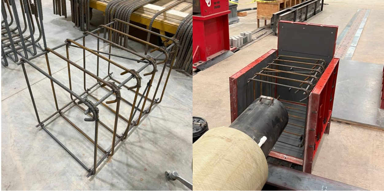
Figure 4-9: Column Cap Components, Rebar Cage (l) and Prefabricated Formwork (r)
