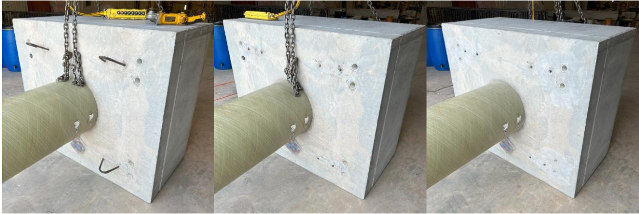
Figure 4-33: Prestressing Strand Lifting Loop Removal and Base Grinding Process
