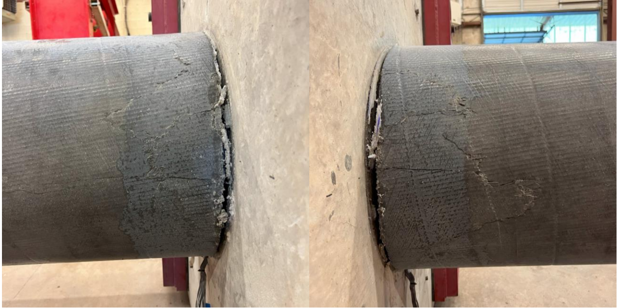
Figure 5-42: UHPC 2 Concrete Core West Side (l) and East Side (r) After Testing
