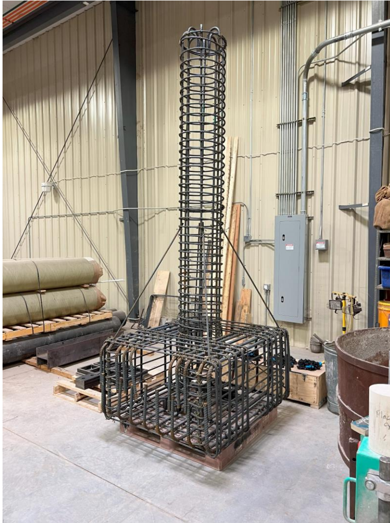
Figure 4-4: Combined RC Column and Base Cages
