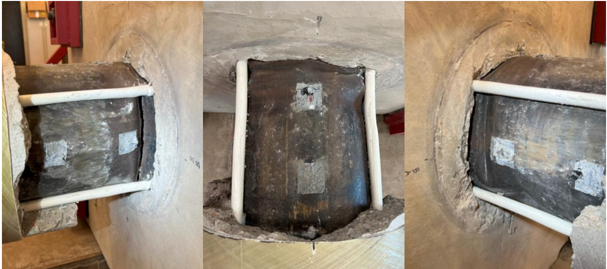
Figure 5-17: HS-SCC 1 Steel Tube West (l), Top (m), and East Side (r) Damage After Testing
