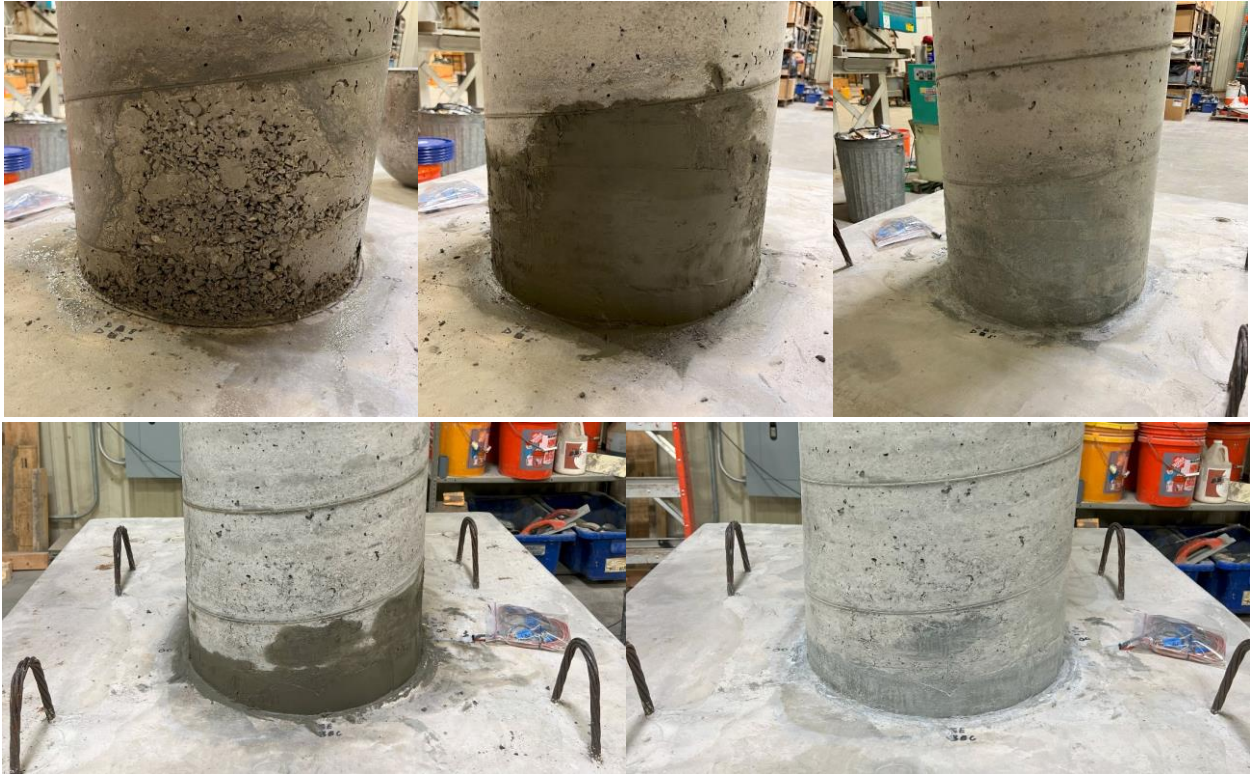
Figure 4-25: RC Column Honeycombing and Cosmetic Patching
