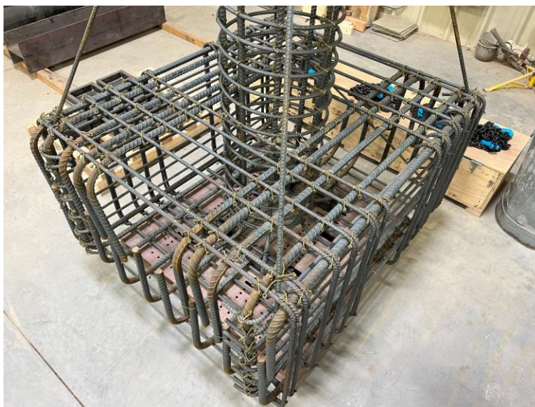
Figure 4-5: Closer Look at the Combined RC Cages
