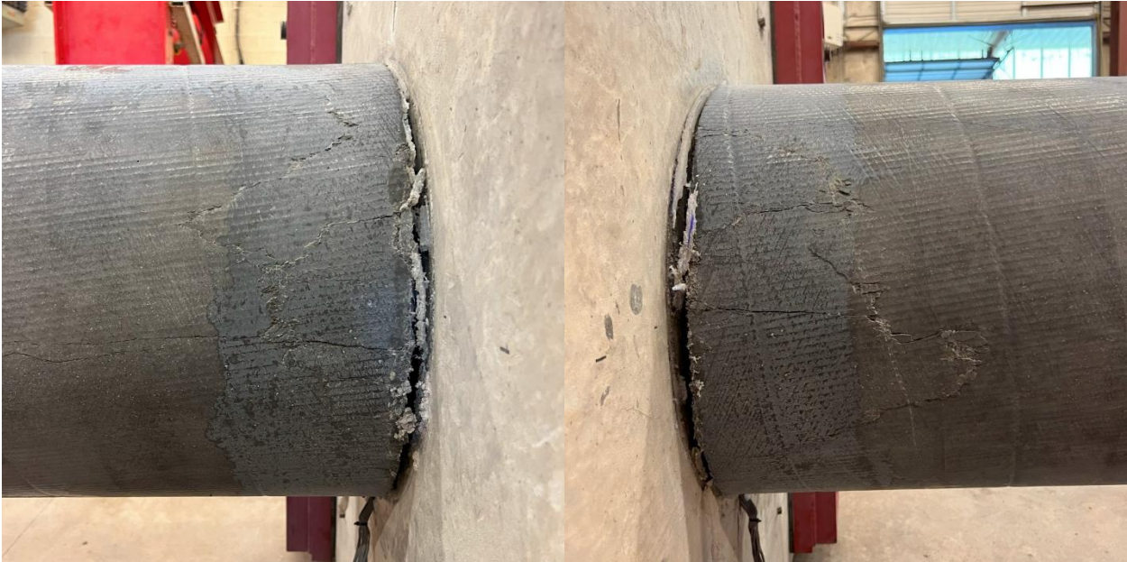
Figure 7-25: UHPC 2 Concrete Core West Side (l) and East Side (r) Damage After Testing
