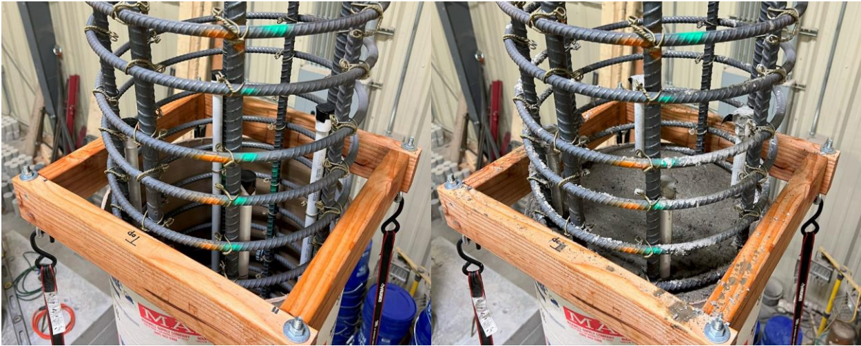
Figure 4-23: RC Column Construction Before Casting and After Casting
