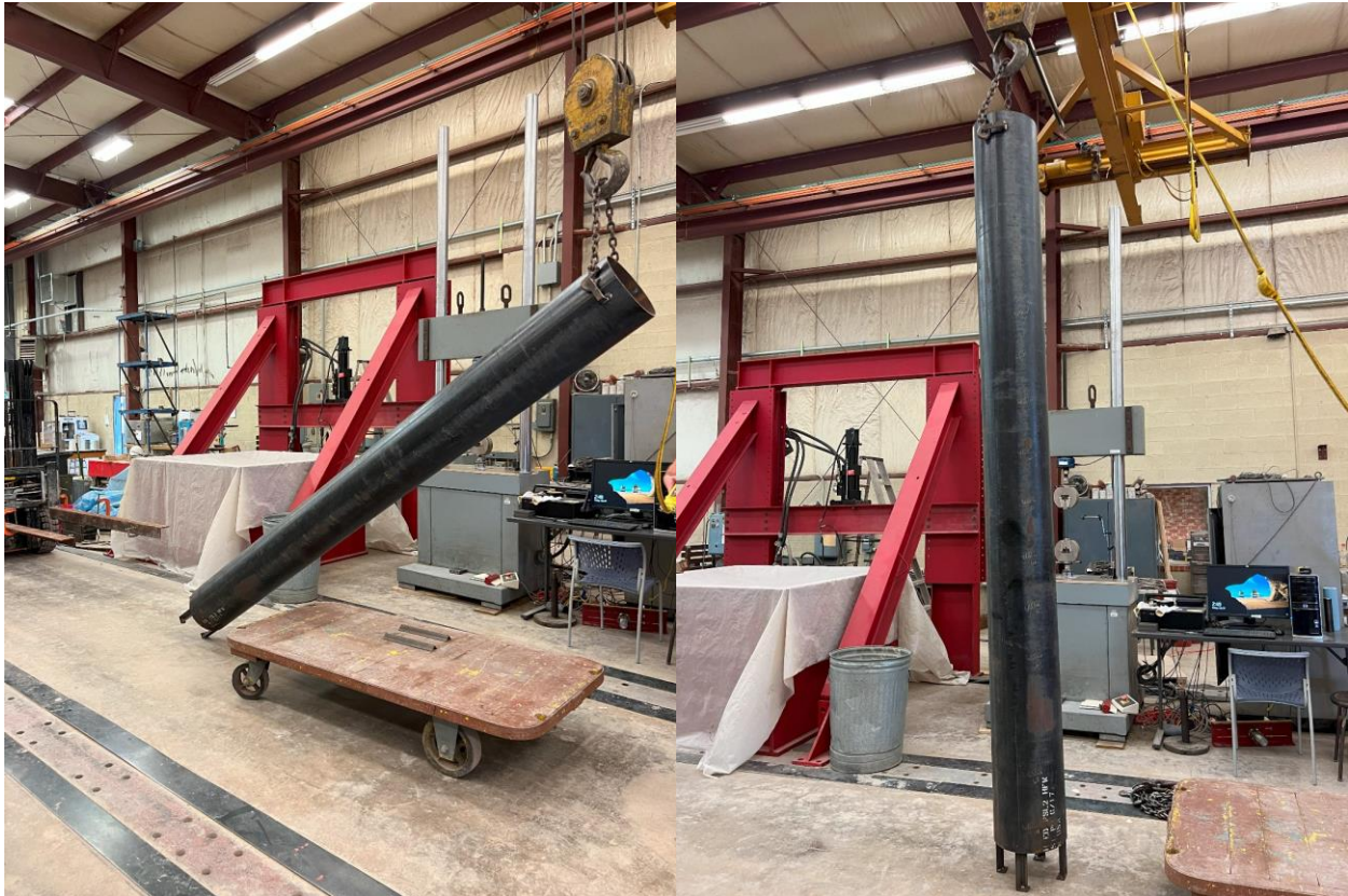
Figure 4-13: Preparing Steel Tubes for Insertion by Tilting Upright with the Crane
