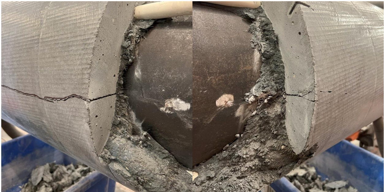
Figure 7-31: UHPC 2 Concrete Core West (l) and East (r) Full-Depth Longitudinal Crack
