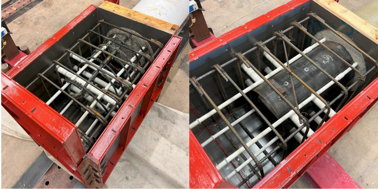
Figure 4-38: Final Column Cap Assembly Before Casting, RC (l) and HC-FCS (r)
