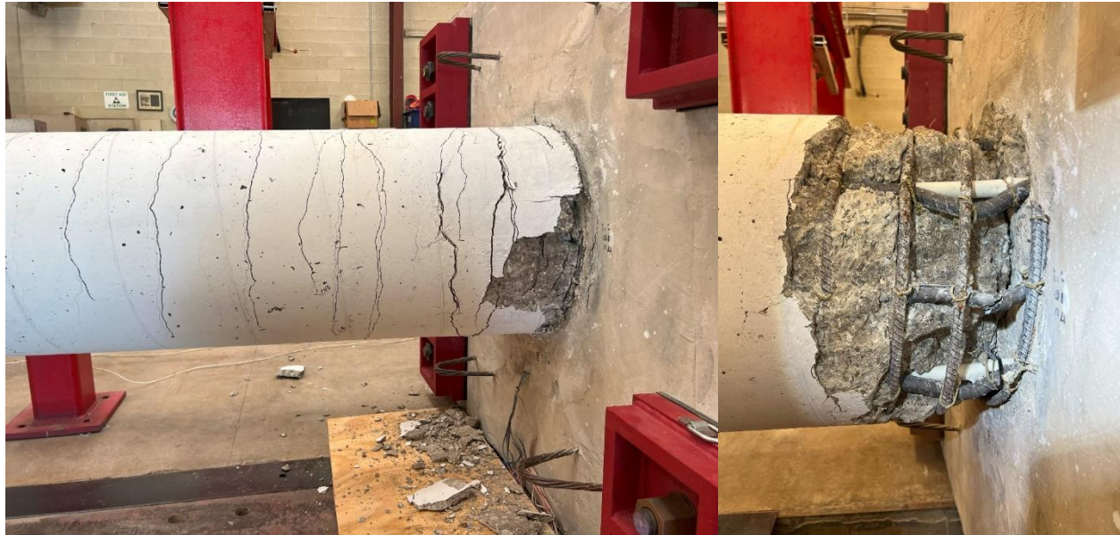
Figure 6-4: RC Column Concentric Circumferential Cracking During Testing (l) and Buckled and Ruptured Longitudinal Bars After Testing (r)
