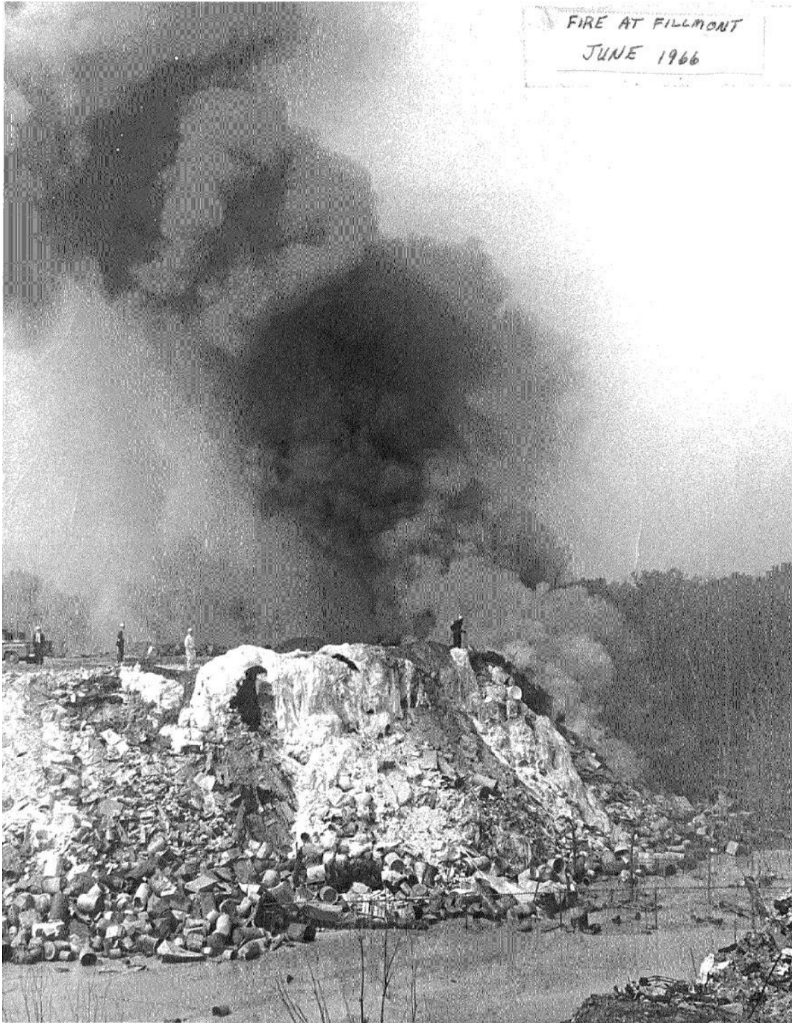
Image 2: Industrial waste on fire at the Filmont Landfill in June 1966.
