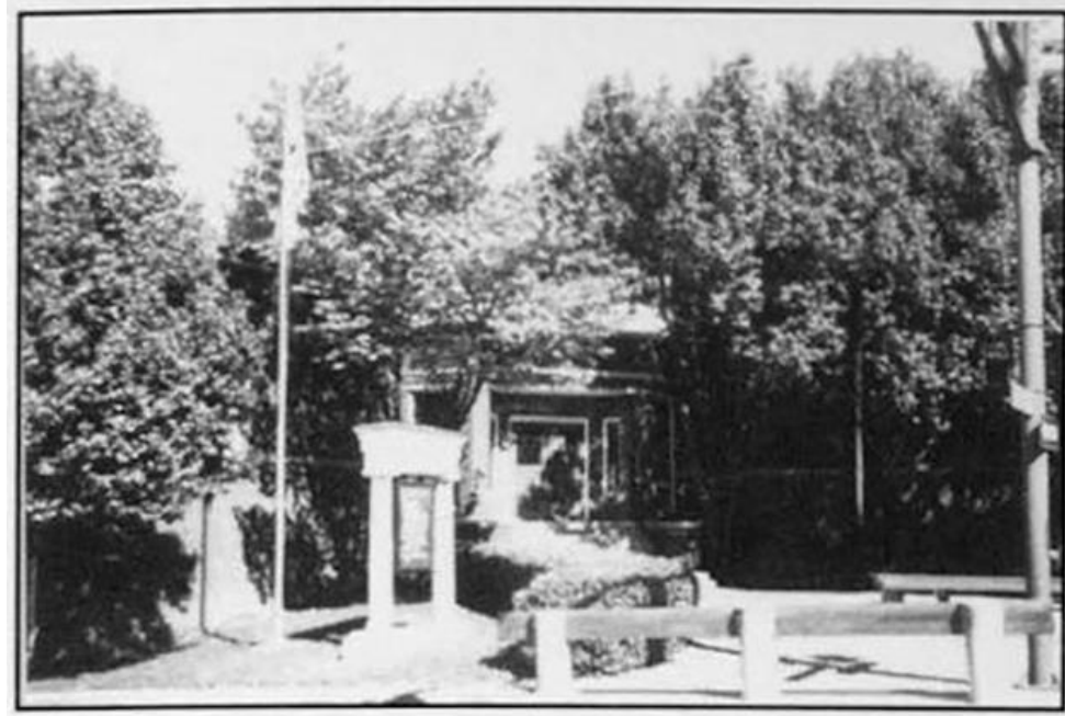
Figure 6: Lee Elementary School (City of Tulsa Preservation Commission, 1996)
