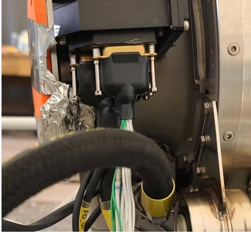
Figure 26. ECU its Wiring Harness.
