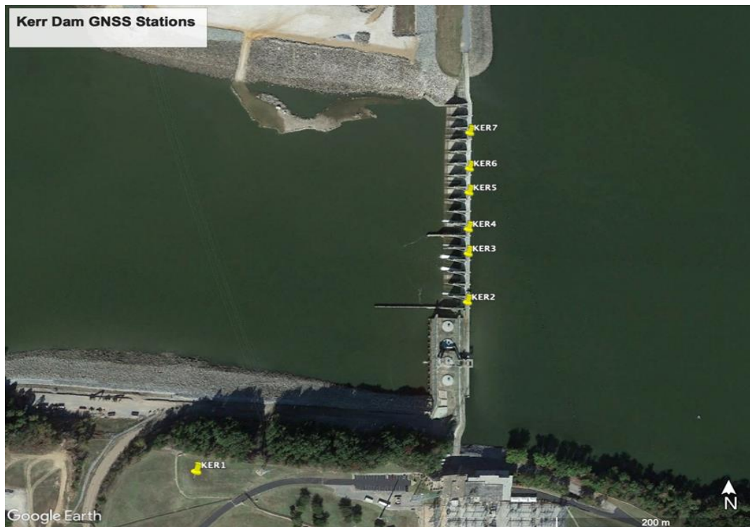
Figure 4: Layout of the stations along Kerr Dam’s crest and reference station KER1.
