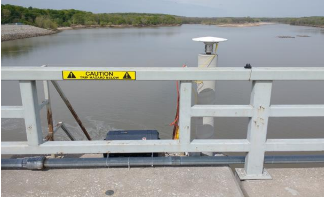
Figure 5: Station configuration of KER4. Each station consists of the Zephyr Model 2 antenna with the Trimble NetR9 receiver stored in a weatherproof Pelican case. Monument is affixed into the structure of the dam.
