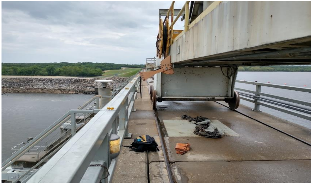
Figure 44: Mobile gate hoist parked near KER3 antenna. Parking hoist near antennas is likely causing signal deterioration from signal reflecting off vehicle and into the antenna. Possible cause of KER5’s poor accuracy.
