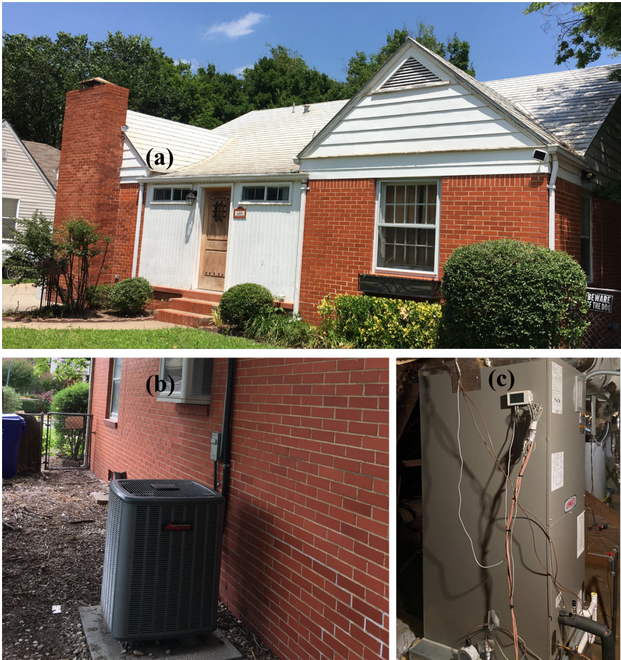
Figure 3.5 Lab House information: (a) outside view of the front of the Lab House (b) an outdoor unit in the back yard of the Lab House (c) an indoor unit in the attic of the Lab House
