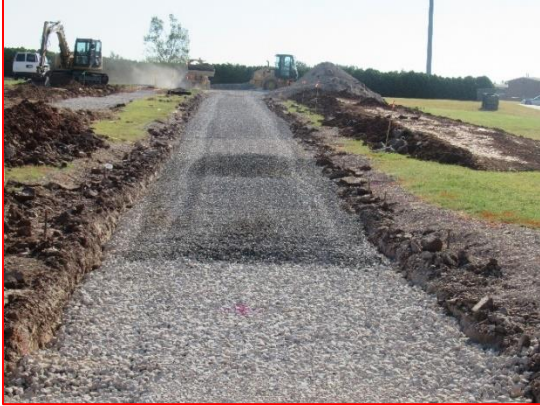
Placement of 4 th Lift (4in ASTM#4)
