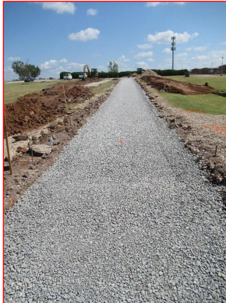
Finished Subbase and Base
