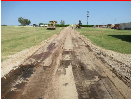
Unprepared Subgrade
