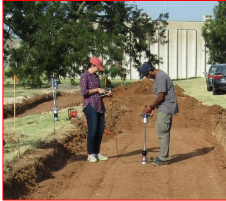
Zorn lab LWD Testing on Subgrade
