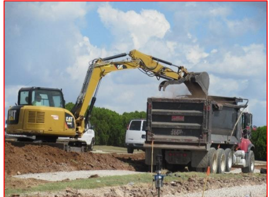
Transportation of the Excavated Soil
