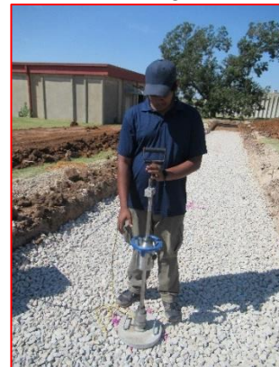
LWD Testing after 3 rd Lift (Olson)
