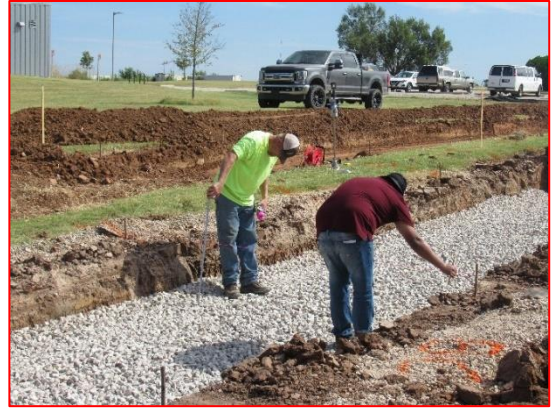
Aggregate Placement and Depth Check
