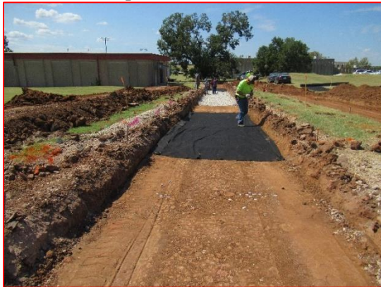
Preparing Other Test cells for Aggregate Placement
