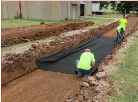
Geotextile Placement
