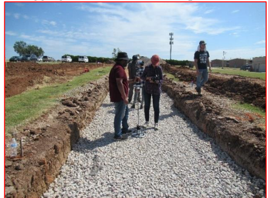
LWD Testing on 1 st Lift after Compaction
