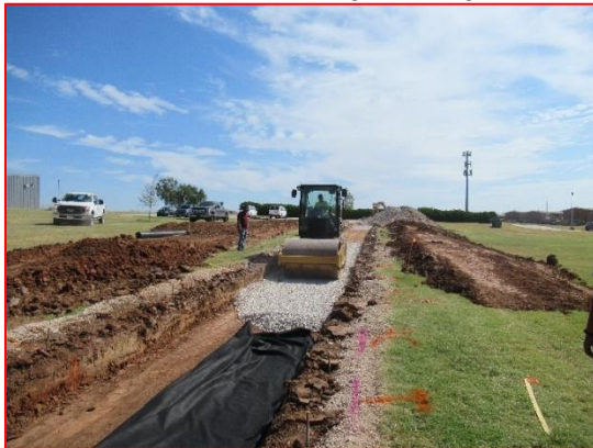
Compaction of 1 st 4in Lift
