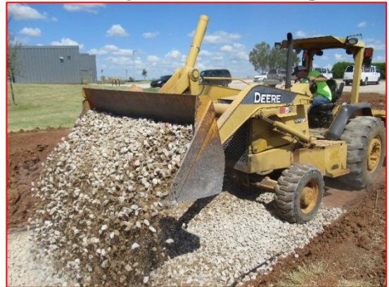
Aggregate Placement
