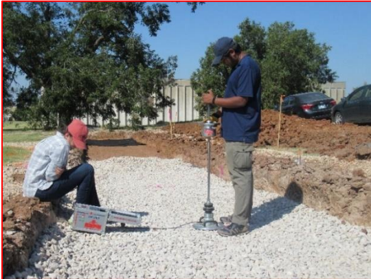
LWD Testing after 3 rd Lift (Zorn)
