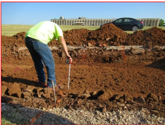
Depth Checking from Baseline
