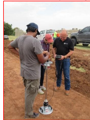
Zorn LWD Testing on Subgrade
