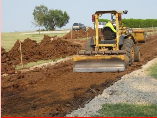
Leveling of Soil by Backhoe Loader
