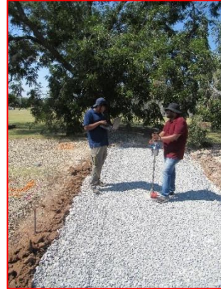
LWD Testing after 4 th Lift and Compacting it
