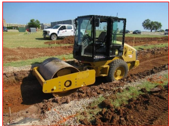
Compacting Subgrade
