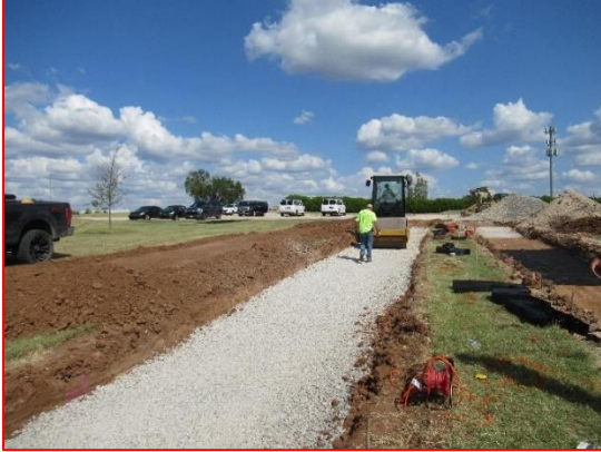
Compaction After 2 nd 6in Lift
