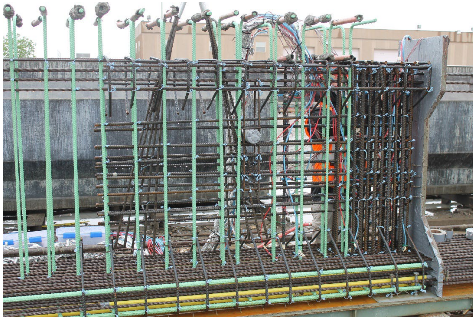
Figure 10: North end reinforcement and instrumentation, Beam Mark 27, Span 9.
