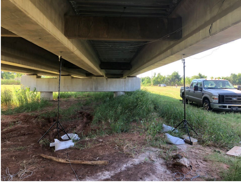
Figure 43: Testing setup for SH 4 load test.
