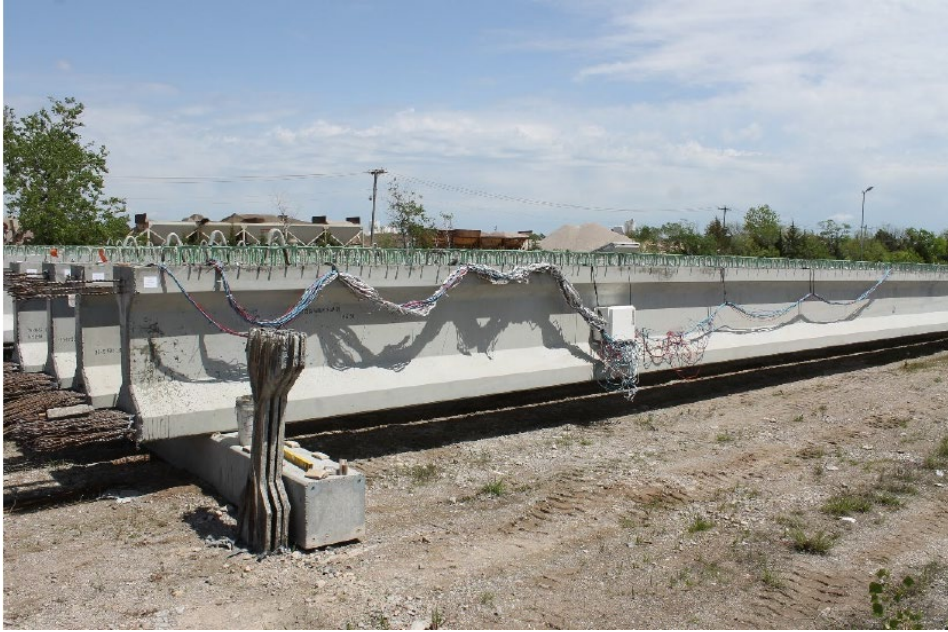
Figure 14: Mark 27, Span 9 at finishing station.
