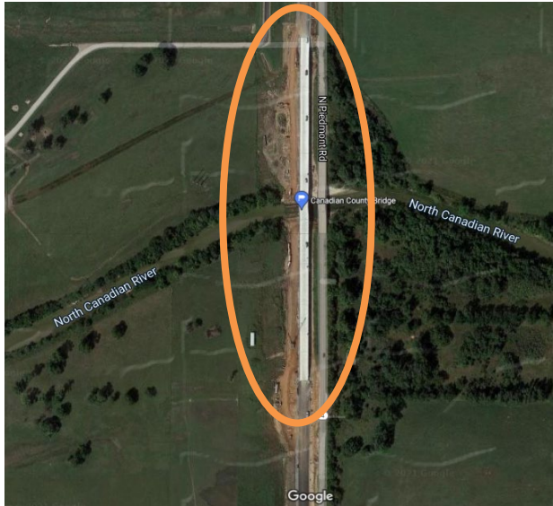
Figure 6: Aerial view of the SH4 bridge over the North Canadian River.
