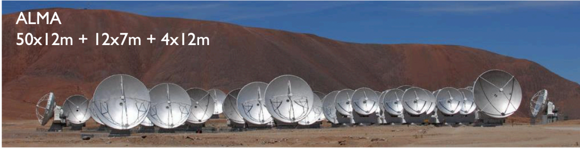
Figure 1.5: The Atacama Large millimeter/submillimeter array, composed of 66 antennas, fifty in the primary, configurable 12-meter array, four in the compact 12-meter array, and twelve 7-meter tertiary antenna. This flexibility in the specific configurations and class of telescopes allows for robust observations that can be tailored to astronomers needs. * credit David. Wilner, Fifteenth Synthesis Imaging Workshop , 2016
