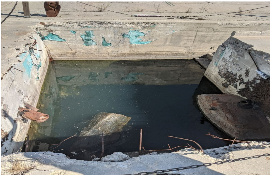
Figure 16 A remaining UST (bottom right corner) found during the October 2022 site visit. Source: (Valerie Doornbos, 2022)
