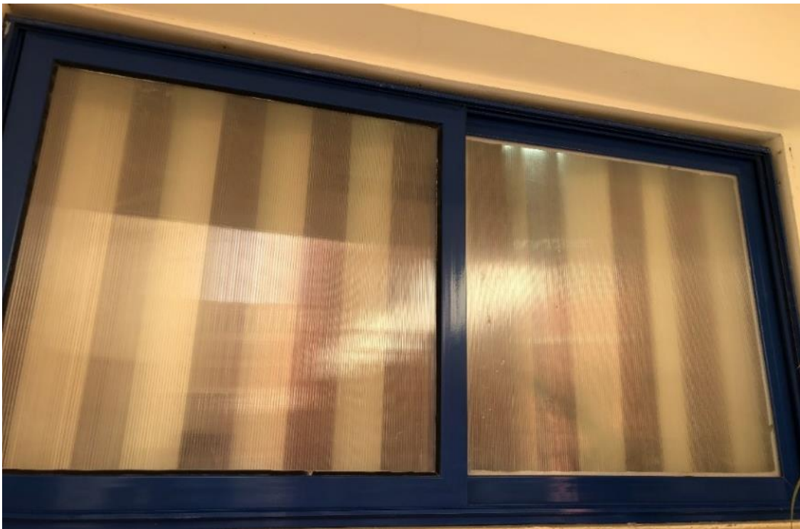
Figure 30. EJS Classrooms windows overlooking main circulation corridors
