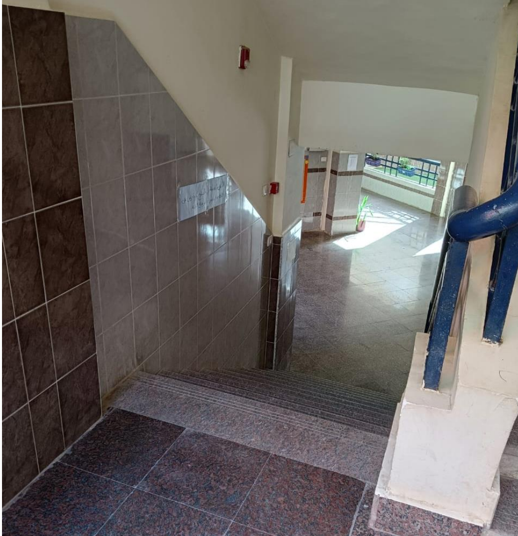
Figure 27. EJS vertical circulation stairs (By: Author)
