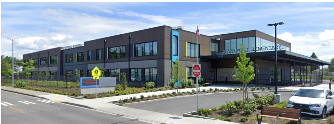
Figure 16. Browns Point Elementary School in Tacoma, WA (Source: Google)
