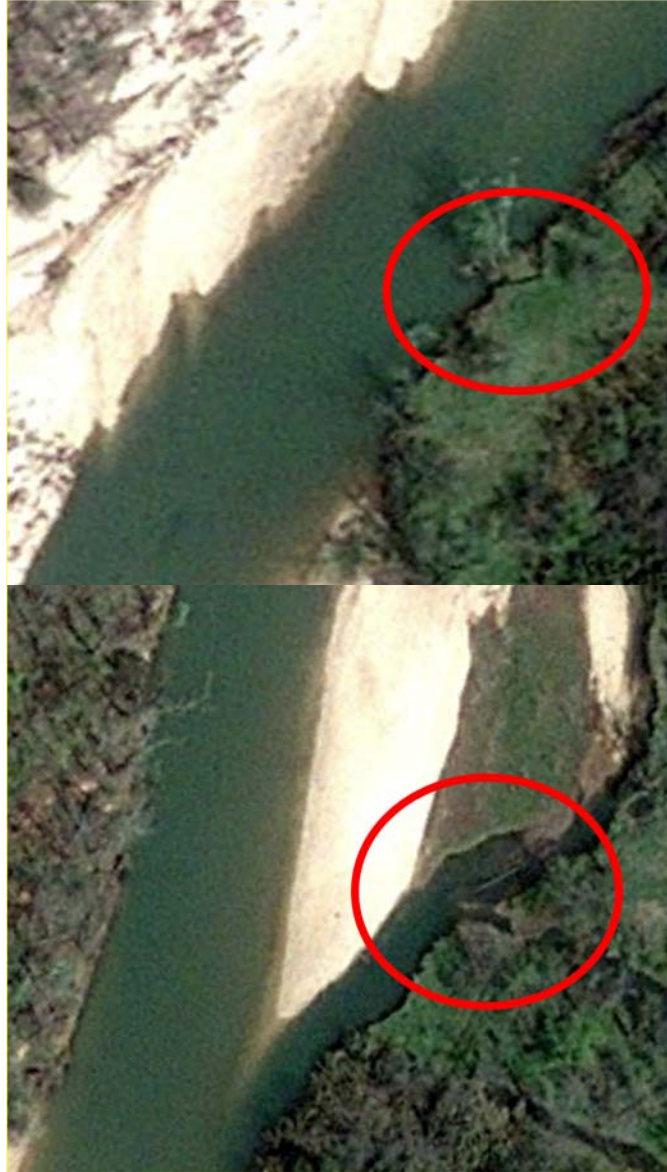
Figure 5: Examples of obvious mass wasting as evidenced by large cracks in the top bank. Google Earth cited both images as coming from DigitalGlobe.
