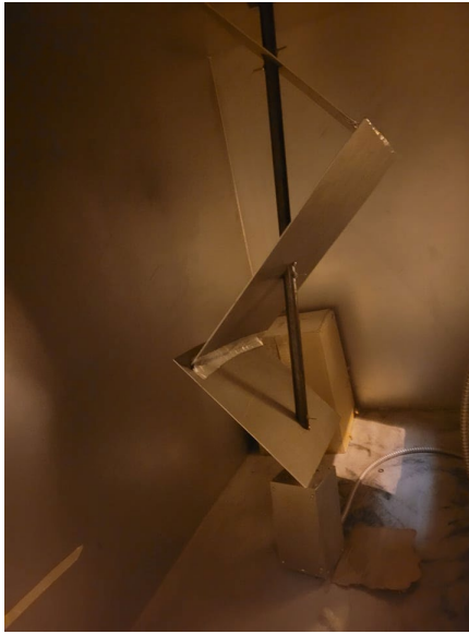
Figure A.4.: Small Chamber Tuner with no aluminum added on to it. (pre-repairs)
