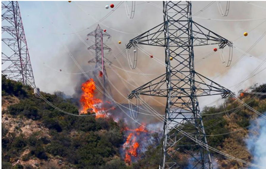
Figure 1: Power Lines Passing through Wildfire affected Area [68]
