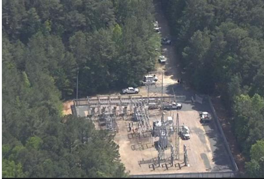
Figure11: Duke Energy Substation located in California Invalid source specified.
