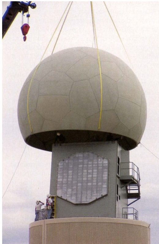
Figure 3.3: NWRT: Installation of the radome over the single aperture of the AN/SPY-IA radar antenna [9].
