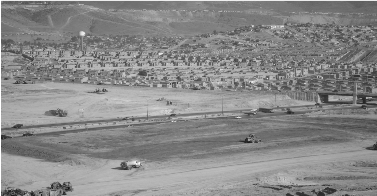
Figure 2 Site preparation for low-income housing construction in the east of Tijuana. 2008
