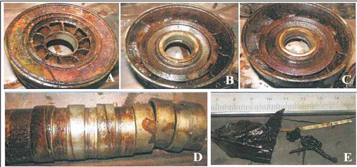
Figure 3-18: Pump Stages Dismantle Findings (Well #2), A) base diffuser's condition, B) middle diffuser's condition, C) head diffuser's wear, D) sleeve's condition at the head, E) debris found in the pump head.
