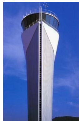
Sondica Airport Tower
