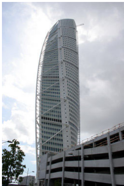
Vertical Bracing System
