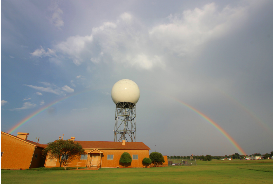
Figure 3.2: Image of KOUN, located in Norman, OK. Photo from Charles Kuster.
