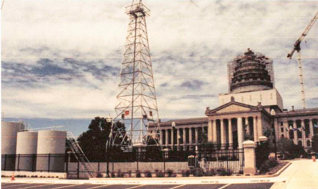
Figure 15 - 2002 Photo of Oklahoma State Capitol building with Petunia #1
