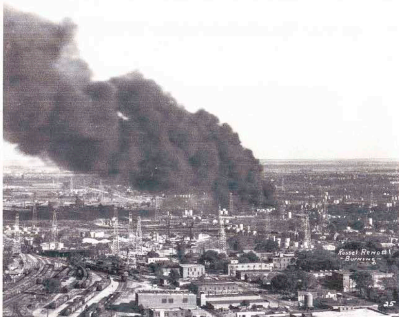
Figure 10 - Oil Well Fire in Oklahoma City Field, Approximate Date 1932
