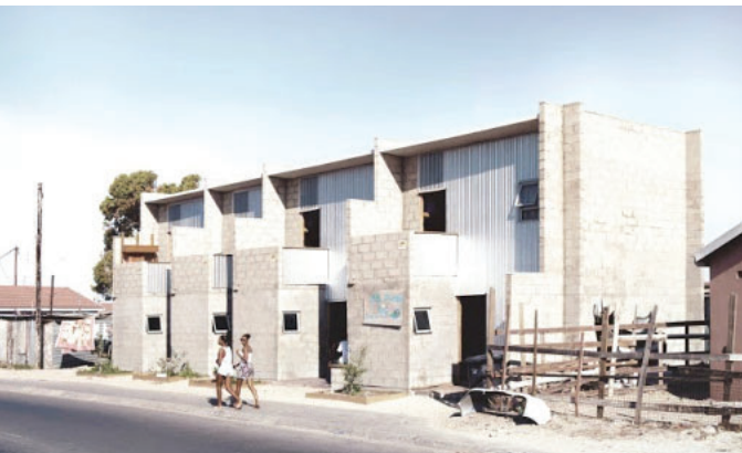
ETH Zurich and Urban-Think Tank partnered with local NGOs to develop four new shacks through reblocking. 12
