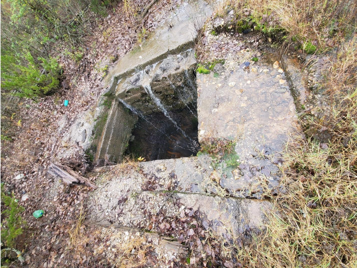
Figure 5B.15: Mid-Continent open mineshaft receiving runoff water during a rain event. Photo taken October 2019
