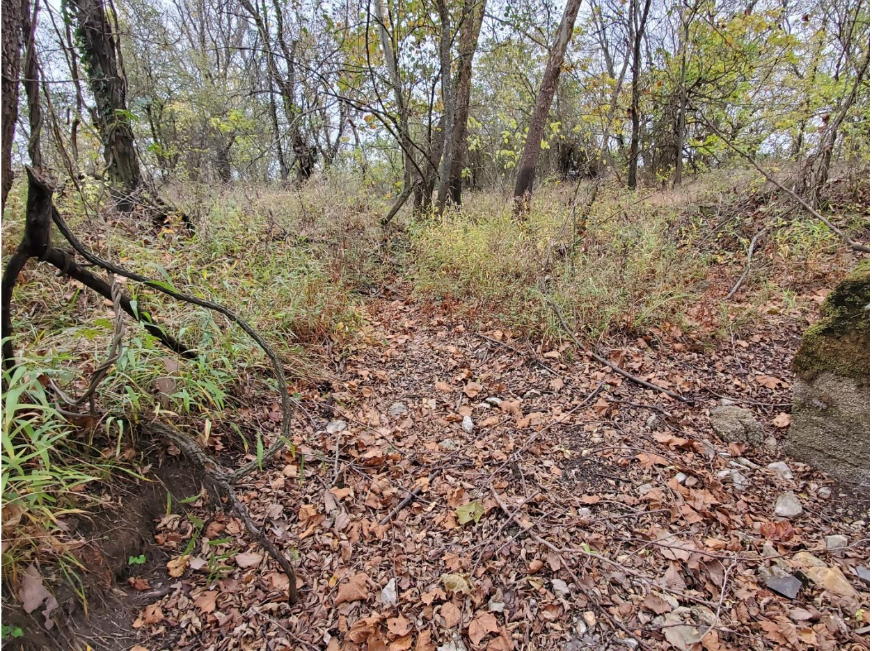
Figure 5B.11: Inflow channel that directs water into the Wesley Smith inflow shaft. Photo taken in October 2020
