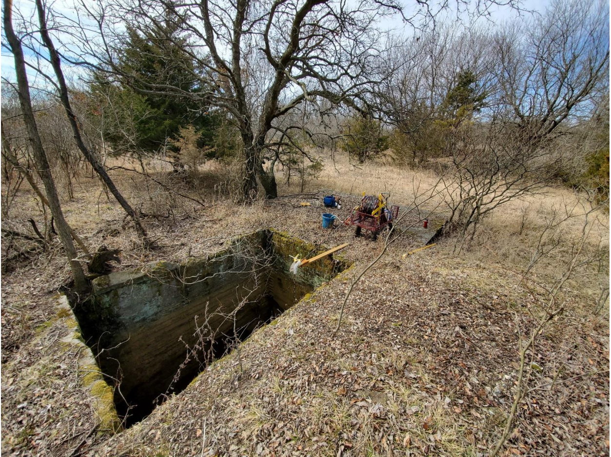
Figure 5B.18: Mary Ann open equipment mine shaft on a typical day. Photo taken February 2021 during a sampling event
