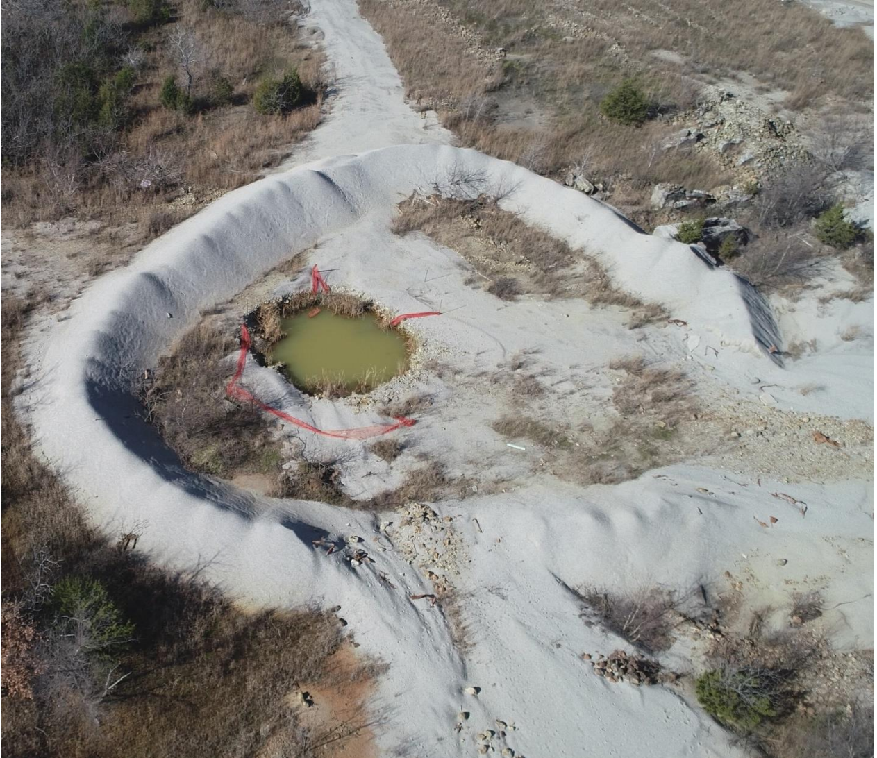
Figure 6B.4: Drone image of the Flint Rock Discharge #2 collapse. Photo taken November 2019 from the north, facing south.
