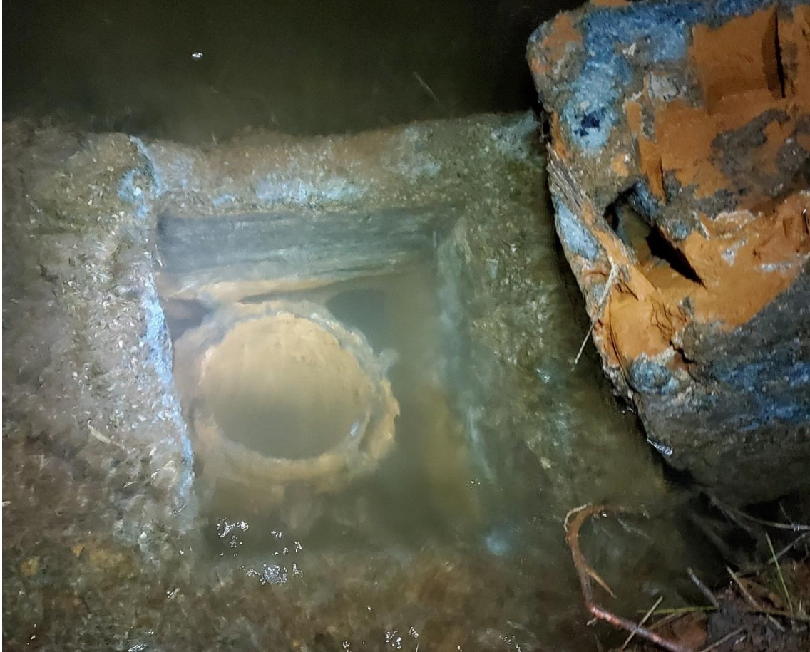
Figure 6A.1: Seep 40 discharge showing the original 10" air ventilation pipe shortly after the concrete cover was removed. Photo taken October 23 rd , 2020
