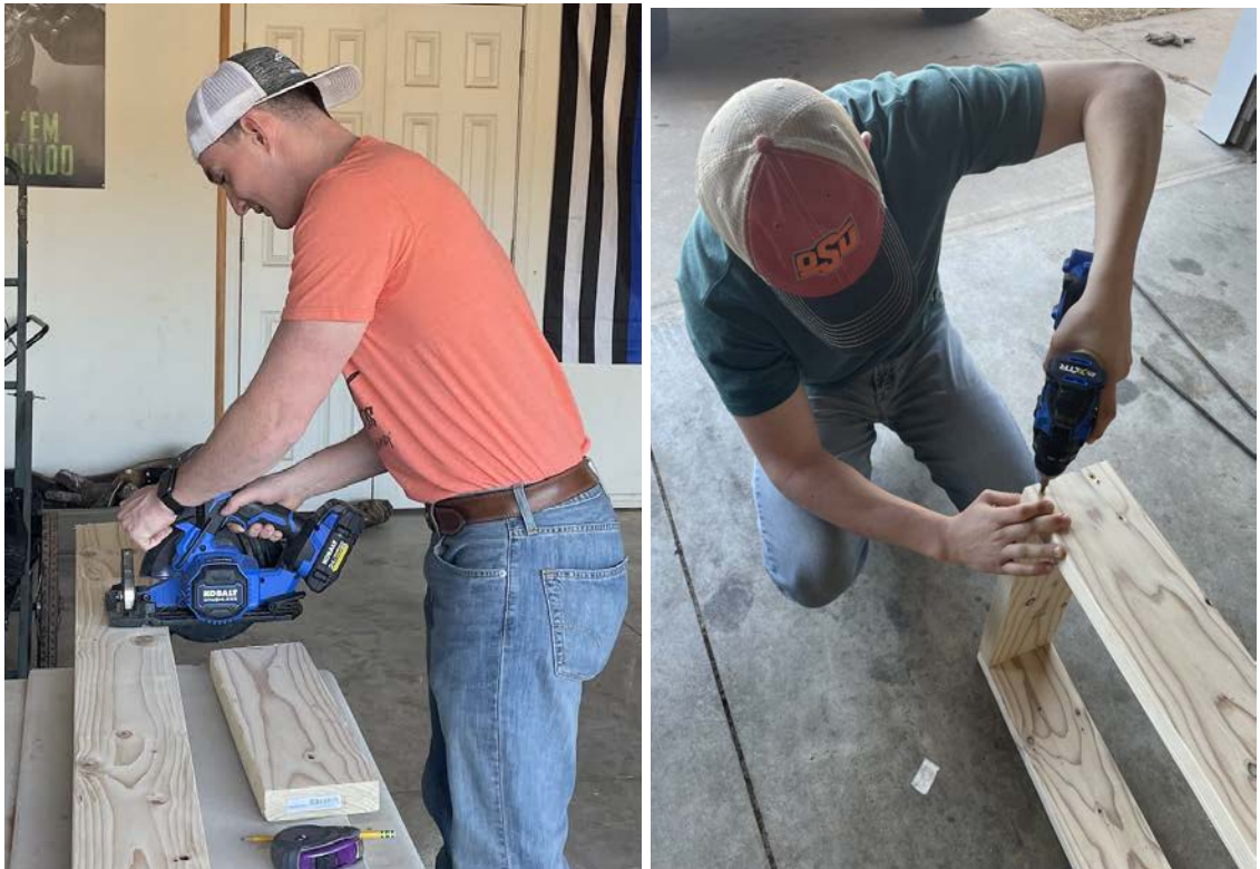
Figure 27. Concrete Mold Construction
