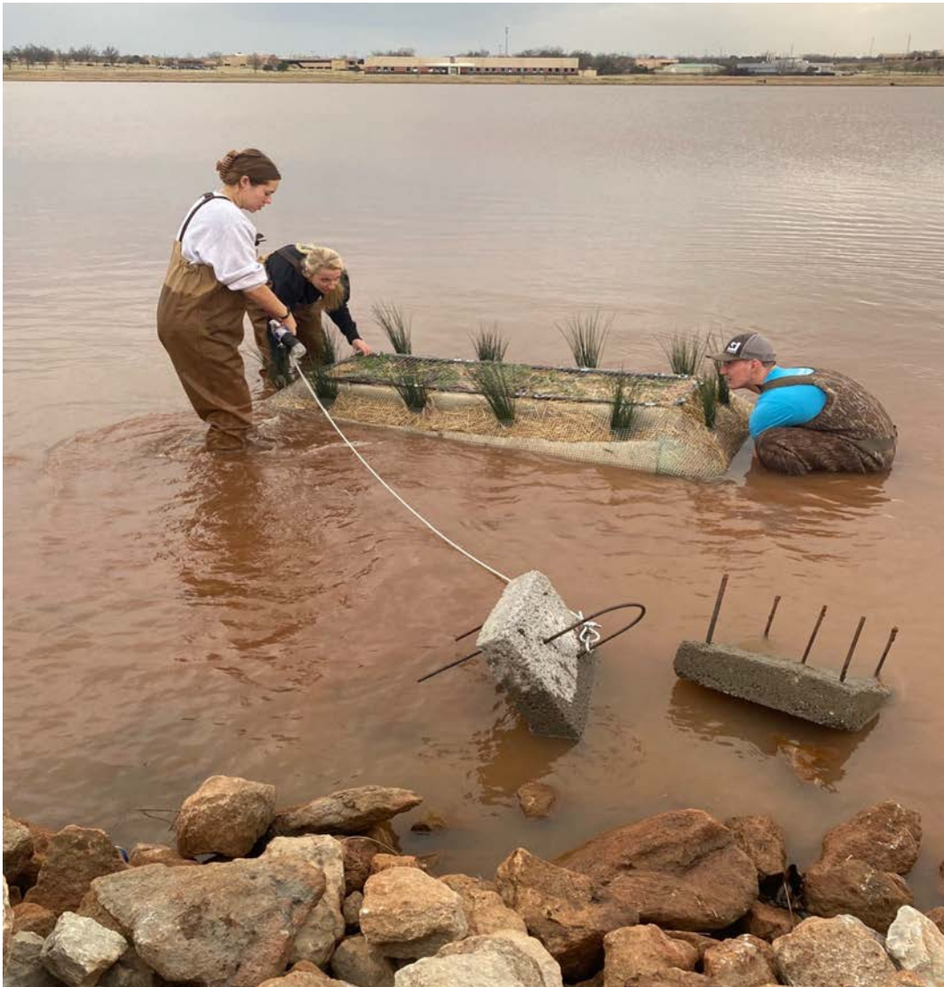
Figure 40. Anchor Cable Attachment
