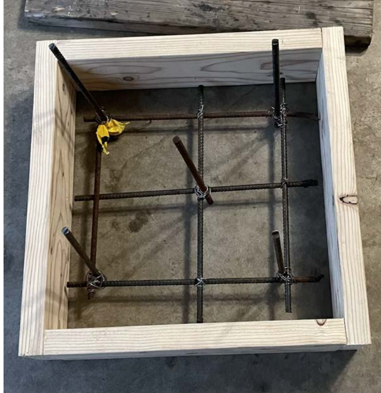
Figure 28. Anchor Construction
