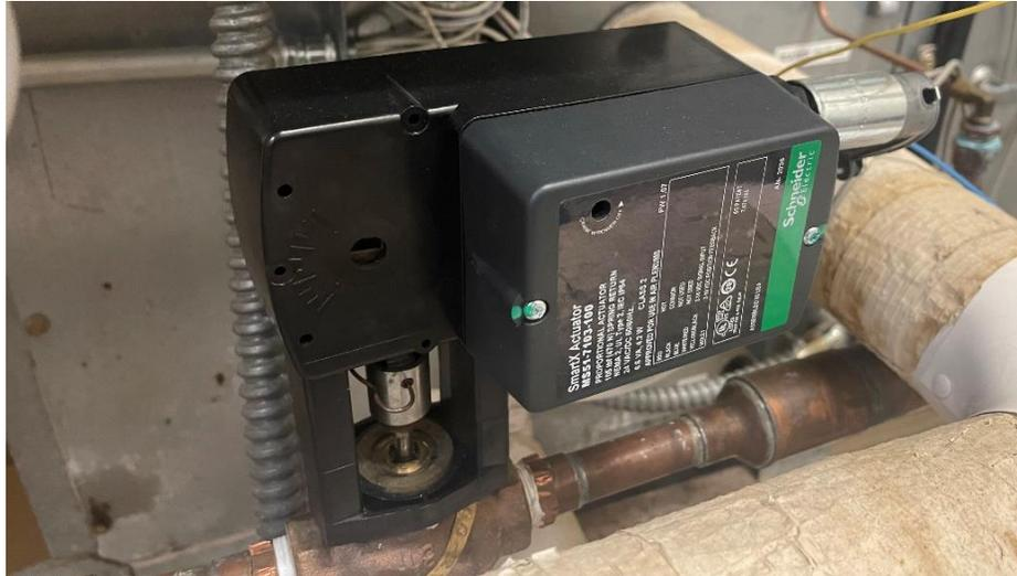
Figure 3-9 The chilled water valve used in the experiment
