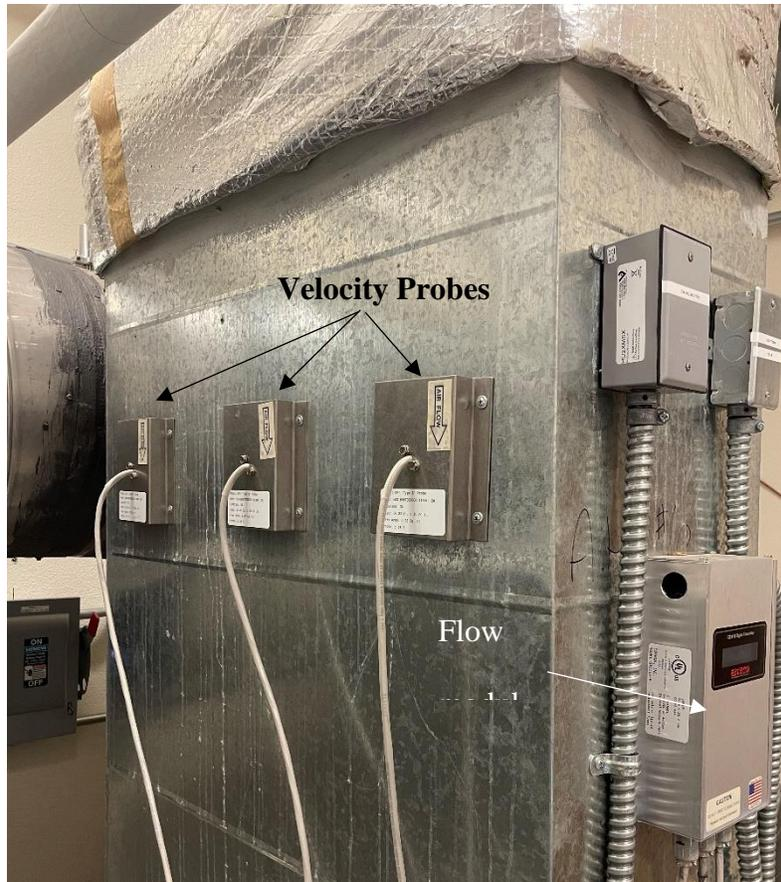
Figure 3-8 Duct Traverse performed for outdoor airflow measurements
