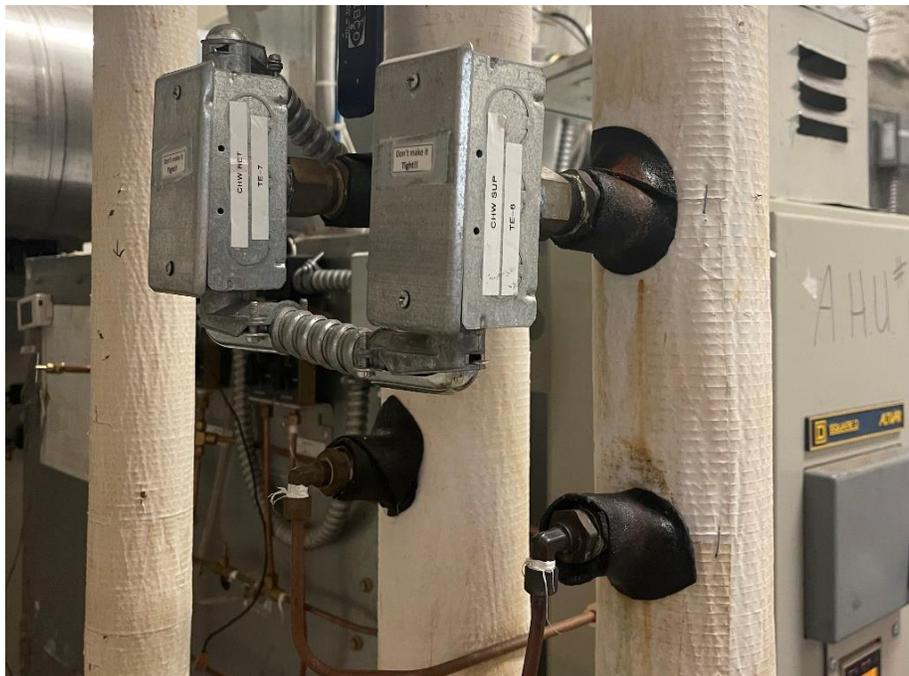
Figure 3-10 Differential pressure sensors installed to measure  $\Delta P_L$
