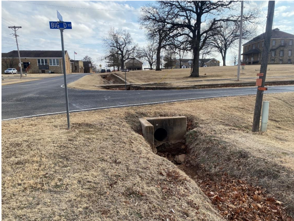
Figure 3: Existing drainage structure at the intersection
