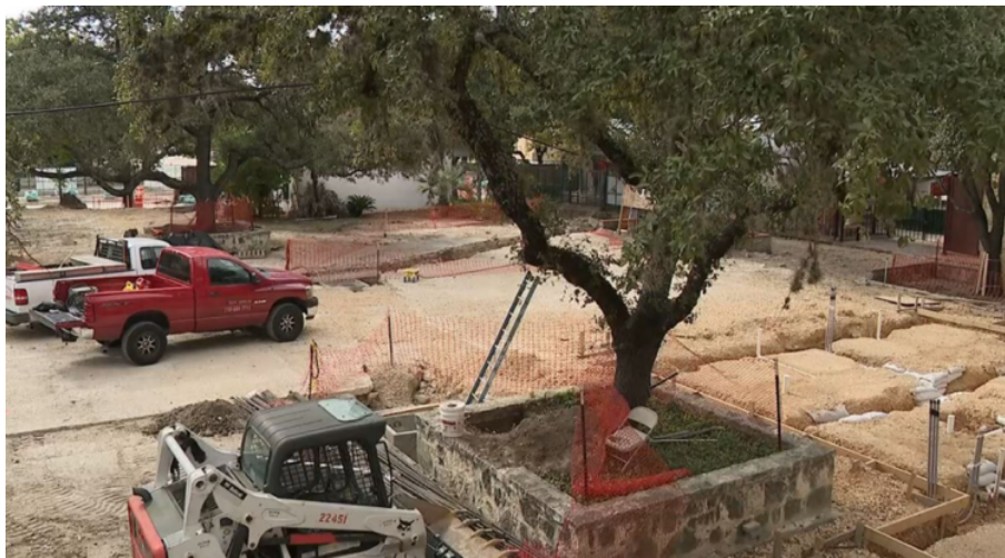
Image 4: Construction Inside La Villita (Sakian)
