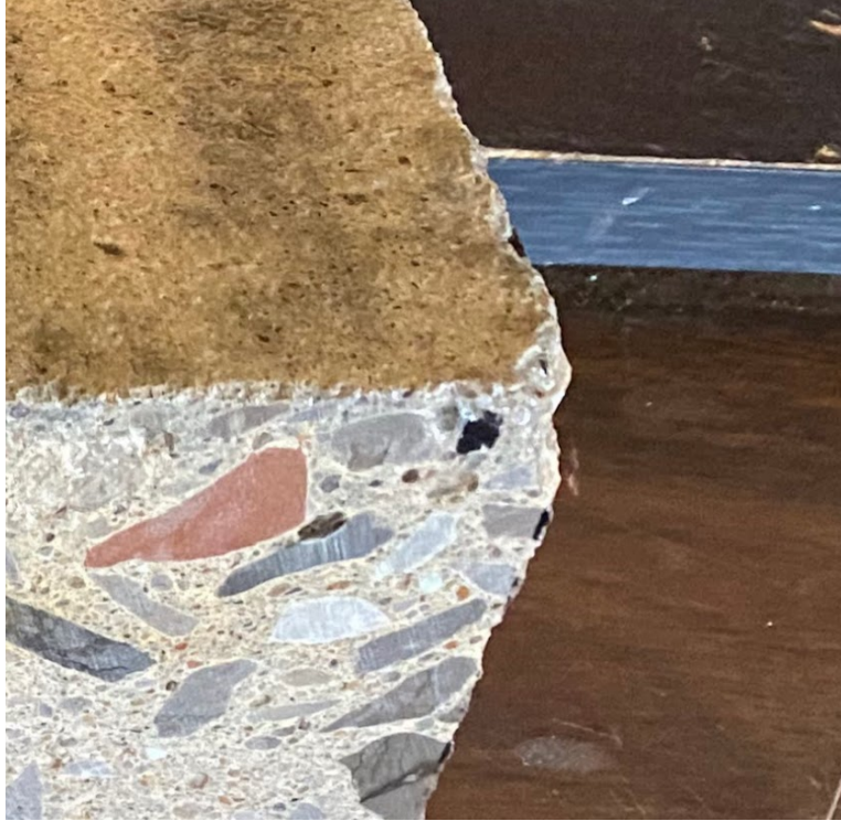
Figure 4-17: Chipped corner of specimen AA2-N
