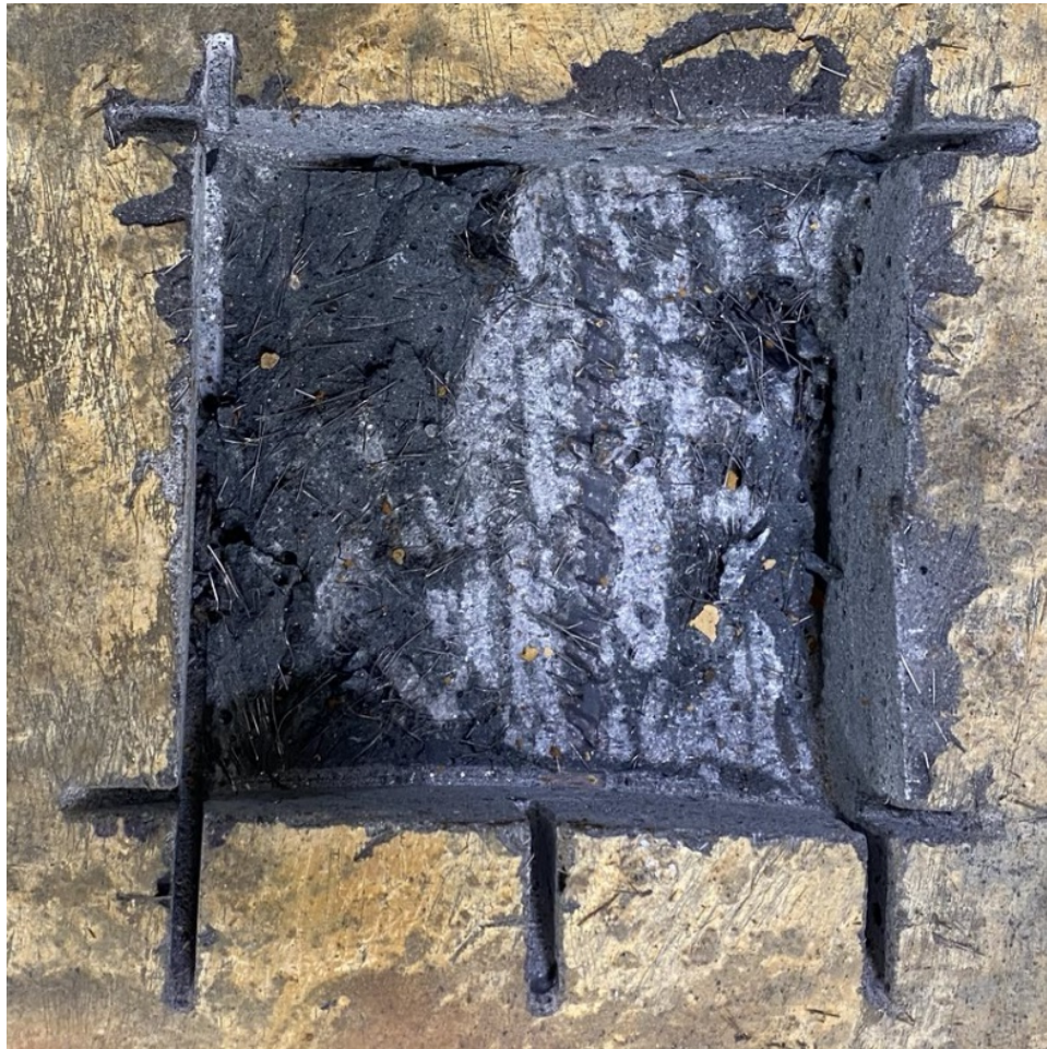
Figure 5-19: CU-N observed rebar A, 37 days tested
