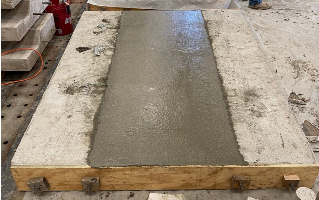
Figure 3-24: Class AA link slab after pouring, leveling
