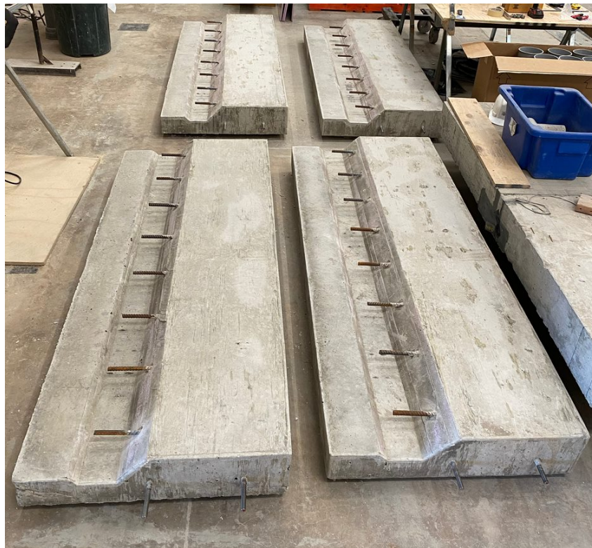
Figure 3-17: Slab sections with foam removed
