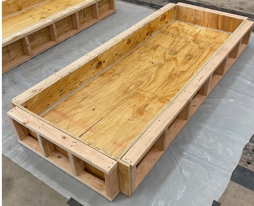
Figure 3-4: Formwork for one slab
