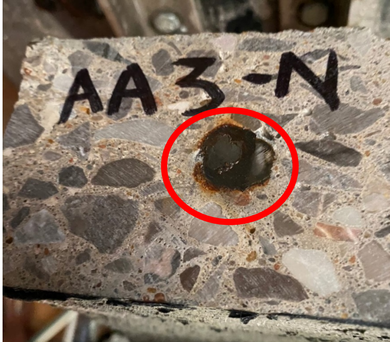
Figure 4-4: End profile of AA3-N with rebar near center (annotated)
