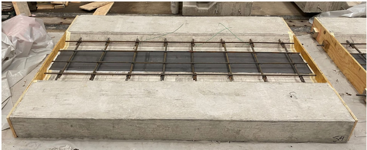
Figure 3-23: Connection fully prepped for casting
