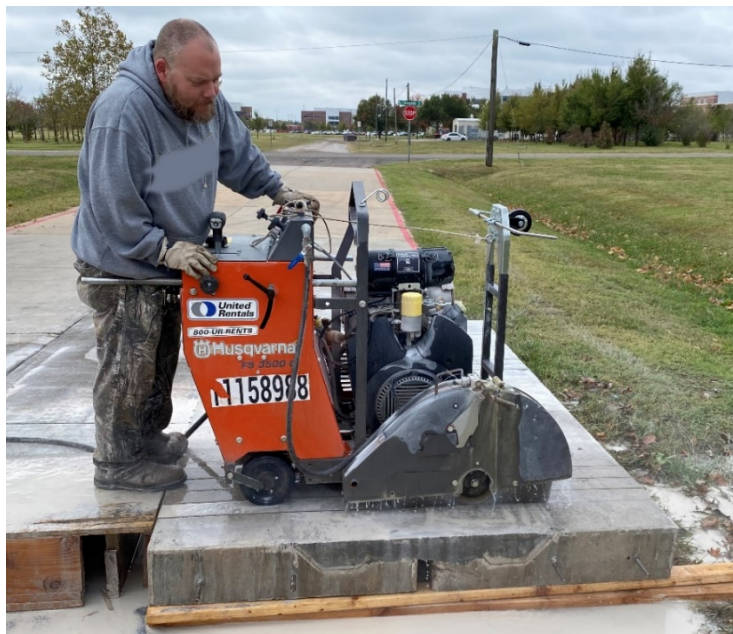
Figure 4-1: Cutting specimen sections from link slab
