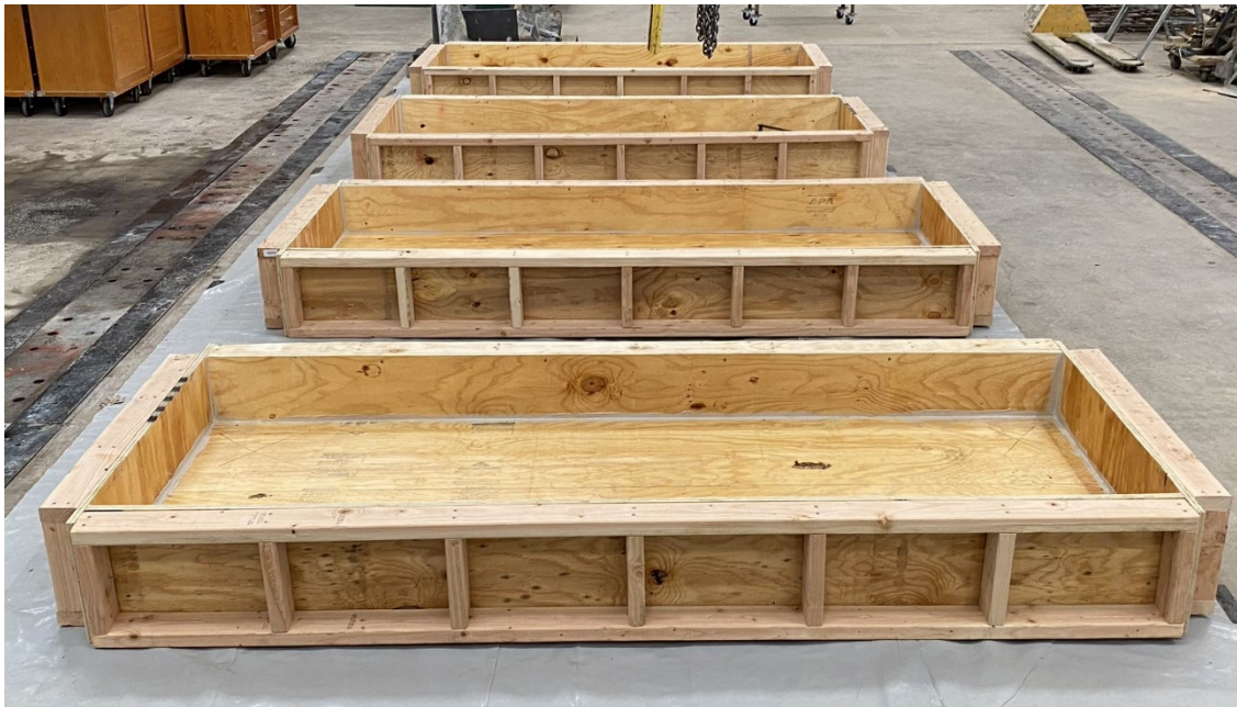
Figure 3-5: Formwork for four slabs
