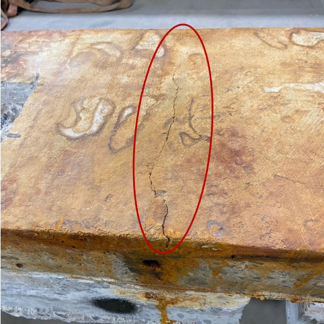
Figure 5-14: Cracking in specimen CAA-N (annotated)
