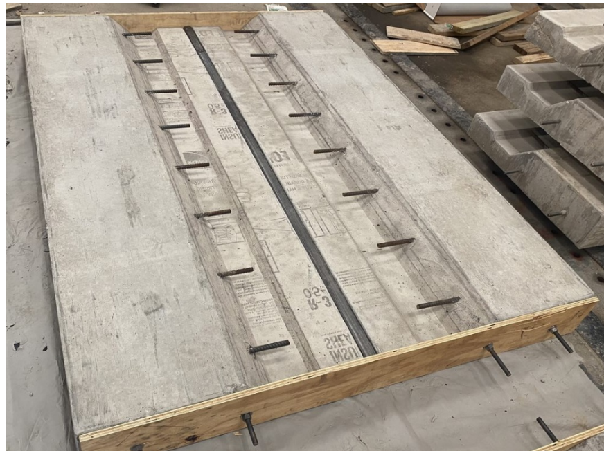
Figure 3-18: Connection preparation with divider, formwork installed
