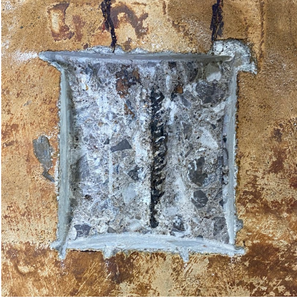
Figure 5-23: CAA-L observed rebar C, 65 days tested
