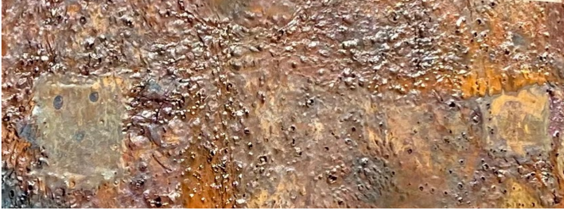
Figure 5-28: Surface of specimen CU-L after 65 days of corrosion testing
