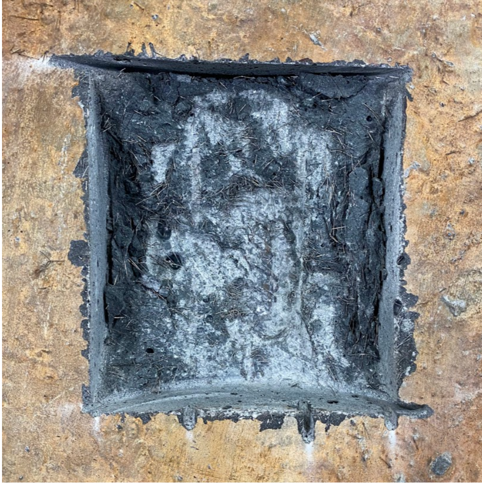
Figure 5-33: CU-N observed rebar D, 65 days tested
