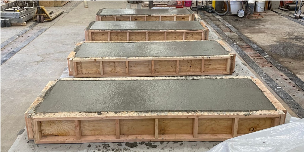
Figure 3-15: Set of slab sections after pouring, screeding
