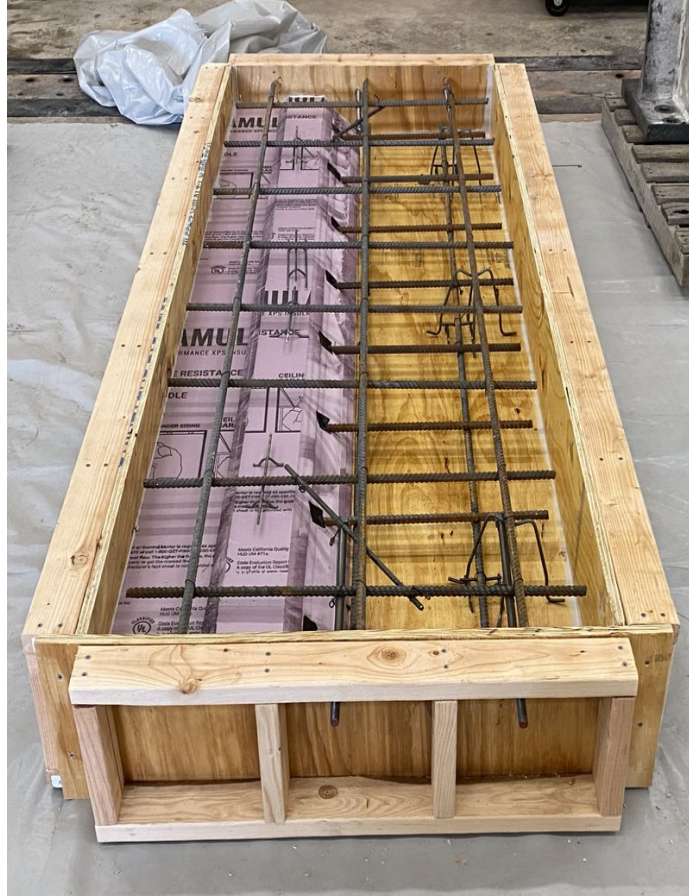
Figure 3-14: Slab formwork with all rebar, all-thread installed
