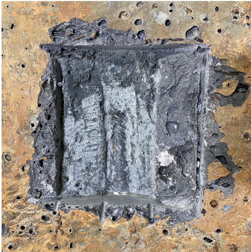
Figure 5-29: CU-L observed rebar C, 65 days tested
