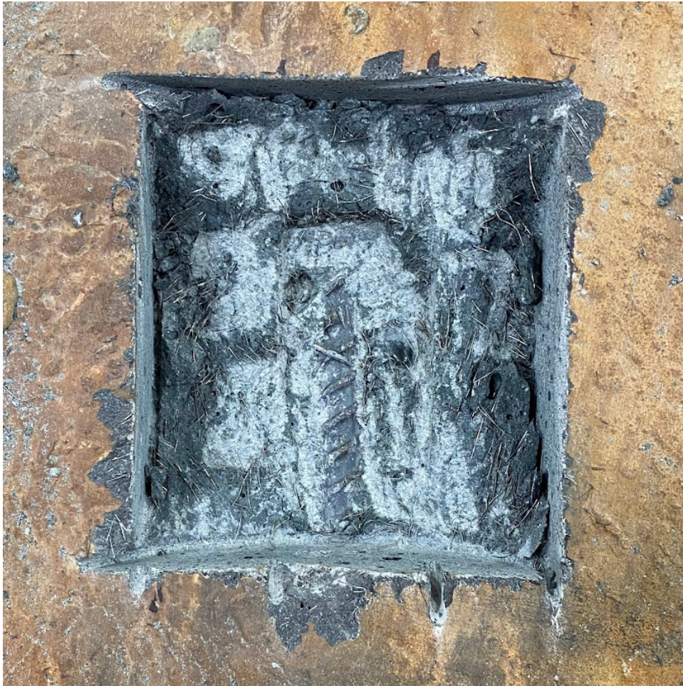
Figure 5-32: CU-N observed rebar C, 65 days tested
