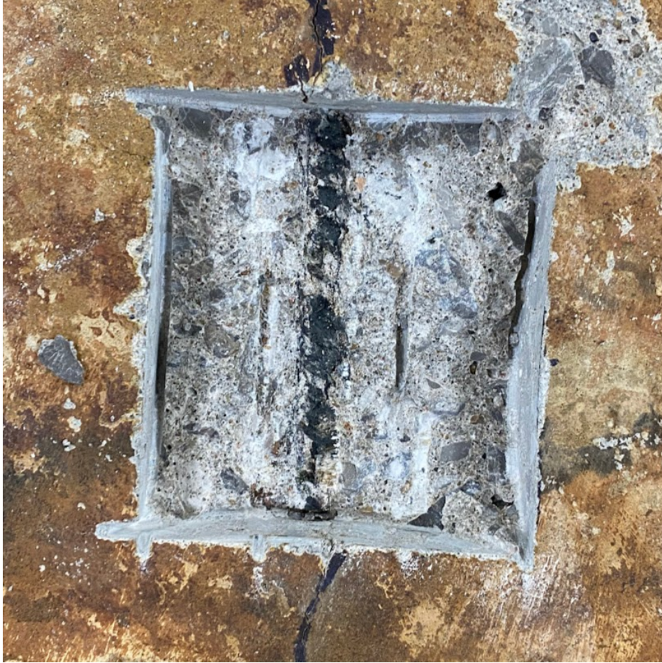
Figure 5-27: CAA-N observed rebar D, 65 days tested
