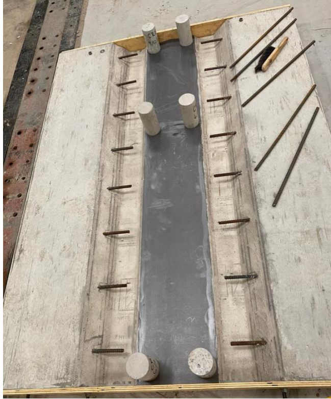
Figure 3-19: Connection preparation with sheet gasket installed
