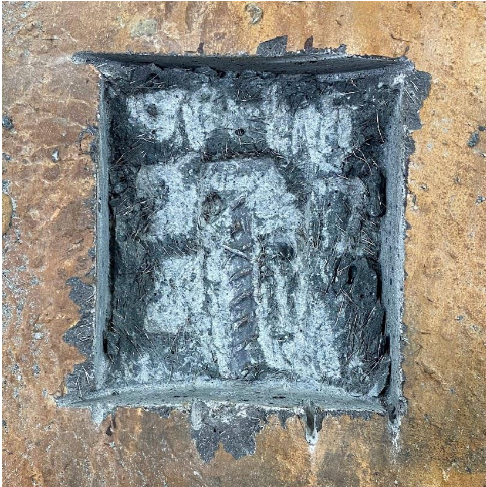
Figure 5-32: CU-N observed rebar C, 65 days tested
