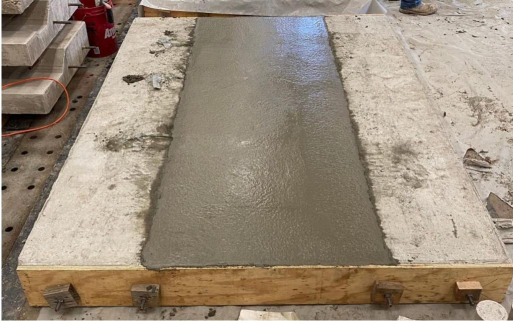
Figure 3-24: Class AA link slab after pouring, leveling
