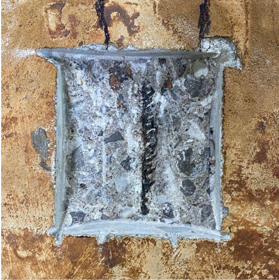
Figure 5-23: CAA-L observed rebar C, 65 days tested
