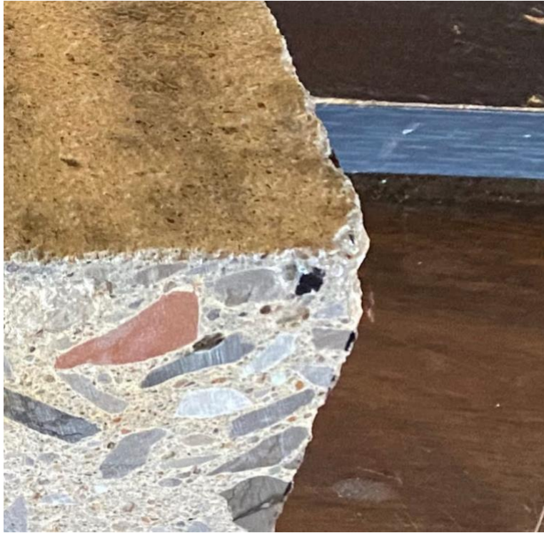
Figure 4-17: Chipped corner of specimen AA2-N
