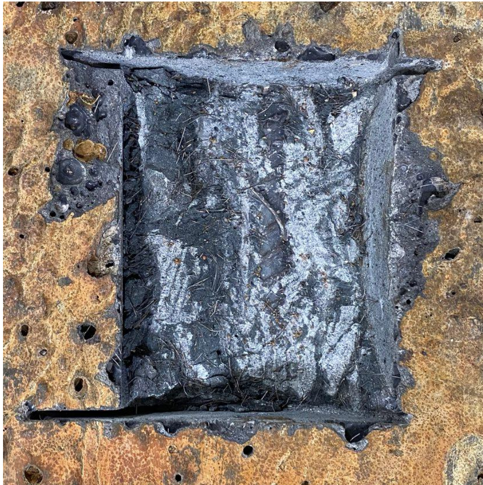
Figure 5-16: CU-L observed rebar A, 37 days tested
