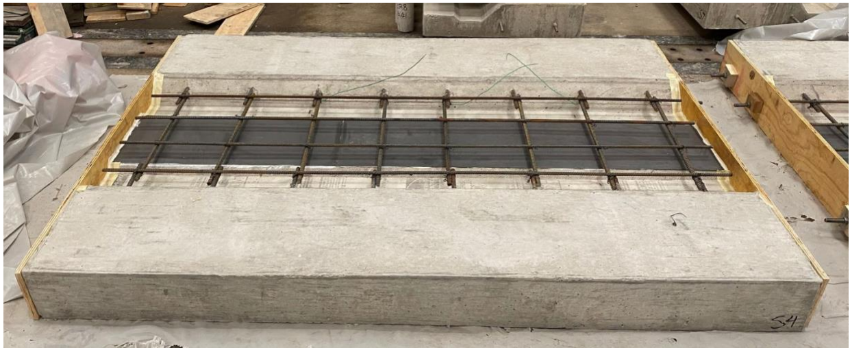
Figure 3-23: Connection fully prepped for casting
