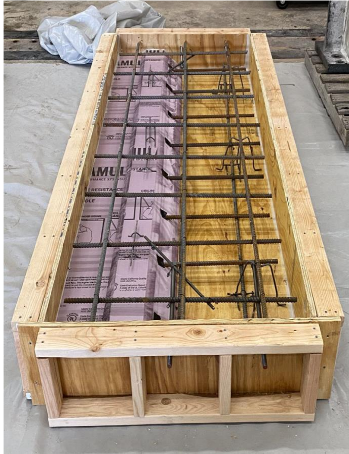
Figure 3-14: Slab formwork with all rebar, all-thread installed
