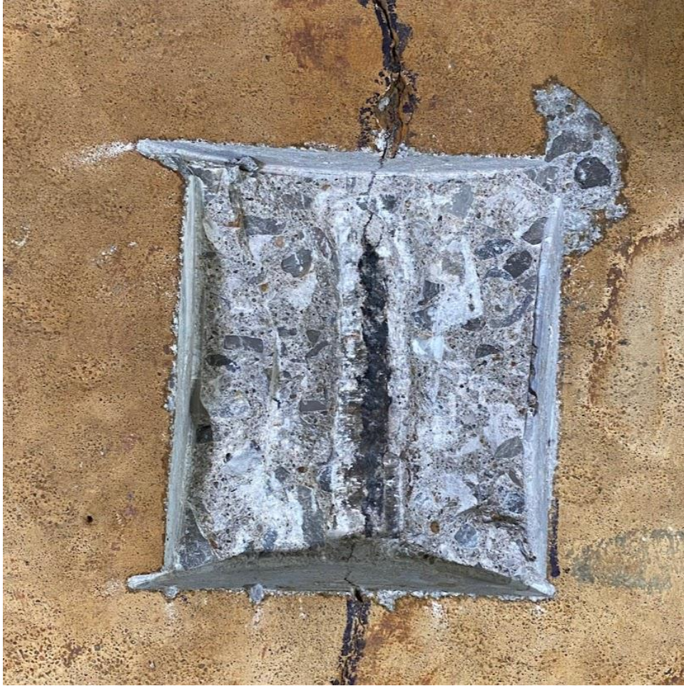
Figure 5-24: CAA-L observed rebar D, 65 days tested
