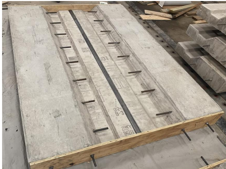
Figure 3-18: Connection preparation with divider, formwork installed
