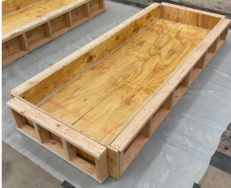
Figure 3-4: Formwork for one slab
