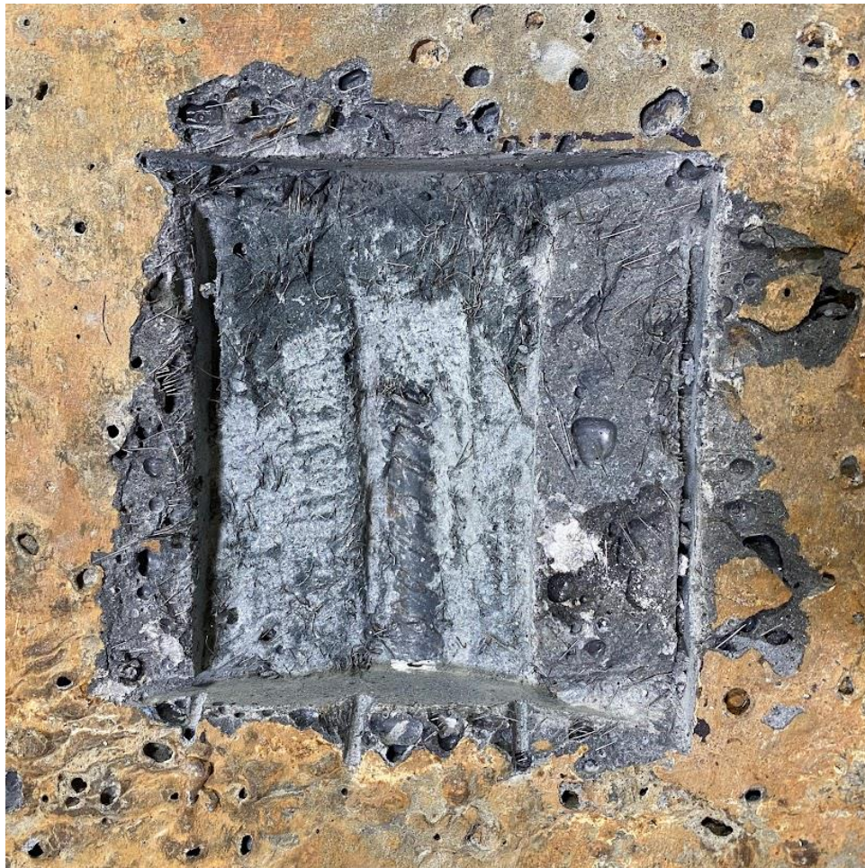
Figure 5-29: CU-L observed rebar C, 65 days tested
