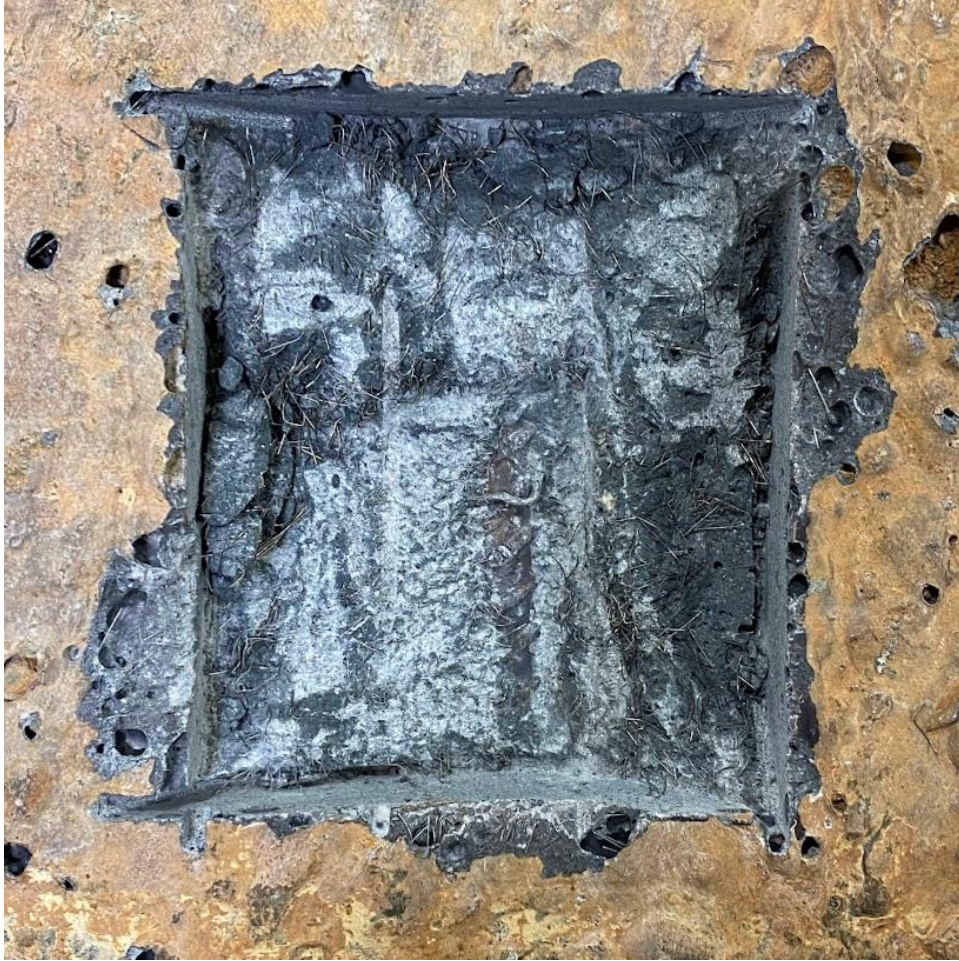
Figure 5-30: CU-L observed rebar D, 65 days tested
