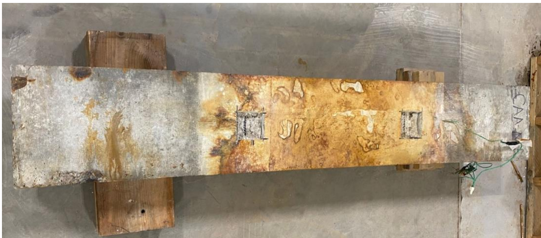
Figure 5-7: Surface of CAA-L after 37 days of testing, windows cut
