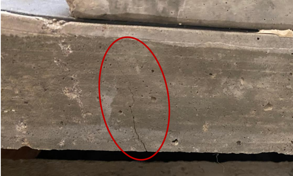
Figure 3-27: Cracking in AA-L during cyclic loading (annotated)
