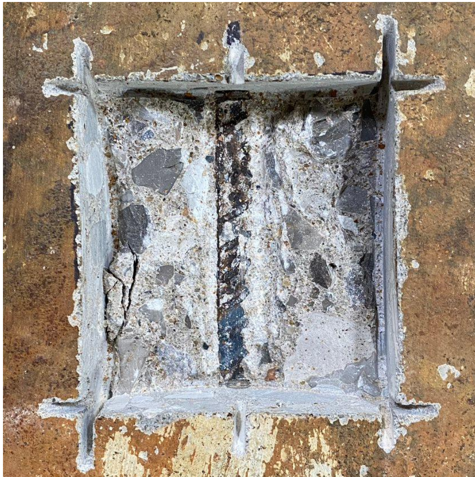
Figure 5-12: CAA-N observed rebar A, 37 days tested
