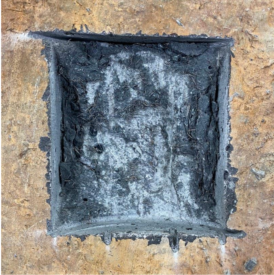
Figure 5-33: CU-N observed rebar D, 65 days tested
