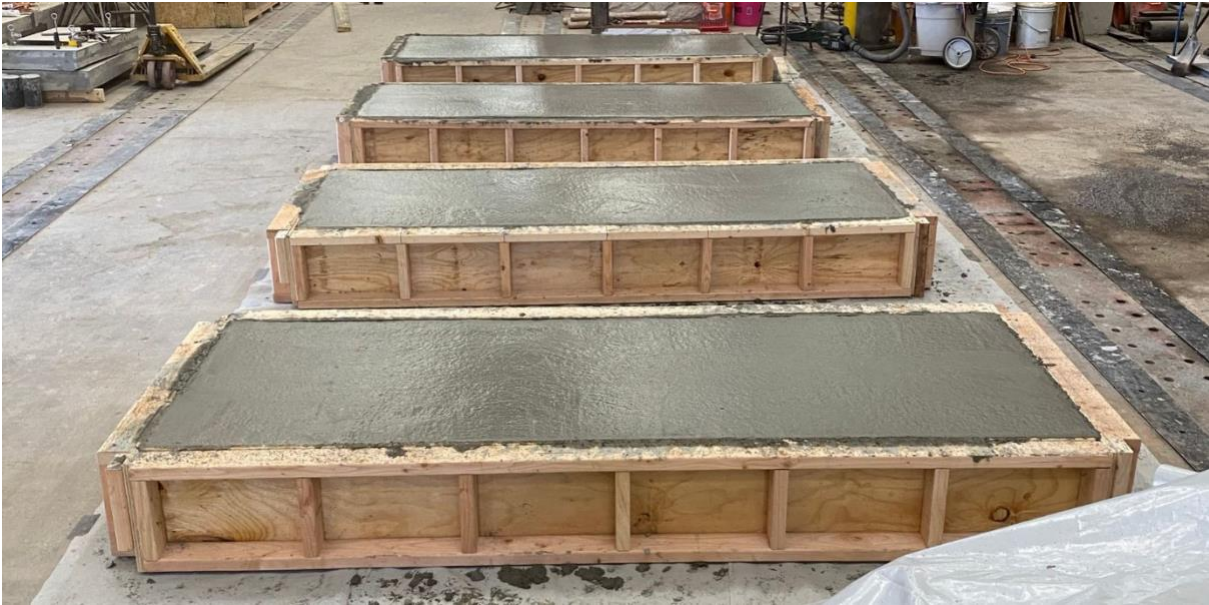
Figure 3-15: Set of slab sections after pouring, screeding
