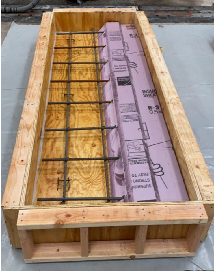
Figure 3-13: Slab formwork with foam insert and "top" rebar cage layer
