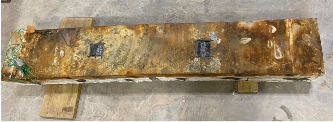
Figure 5-18: Surface of CU-N after 37 days of testing, windows cut
