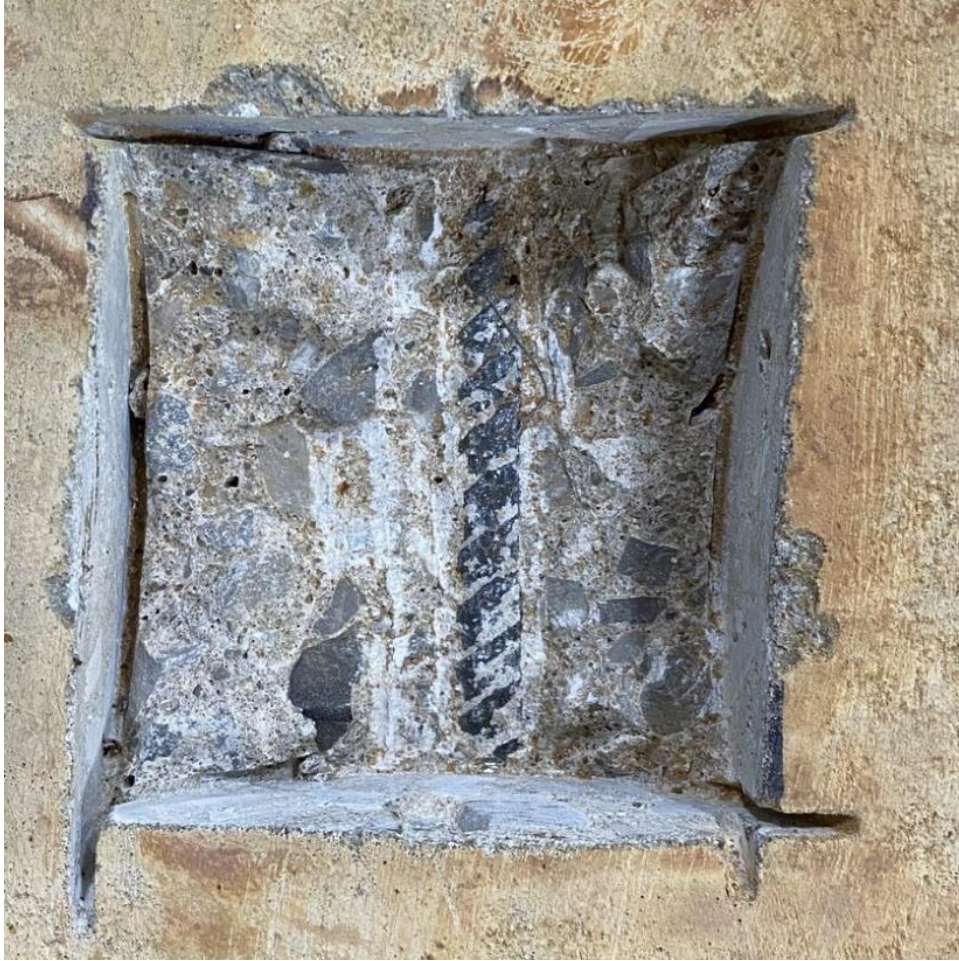
Figure 5-9: CAA-L observed rebar B, 37 days tested
