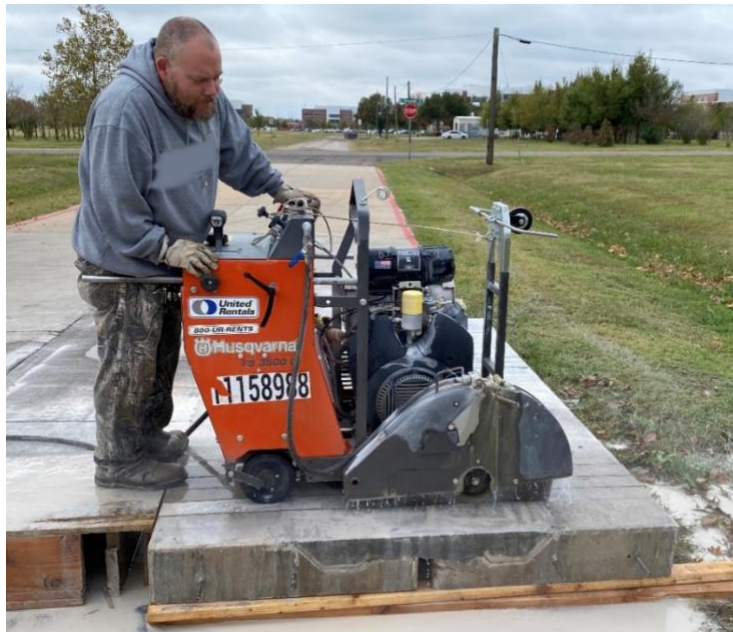
Figure 4-1: Cutting specimen sections from link slab
