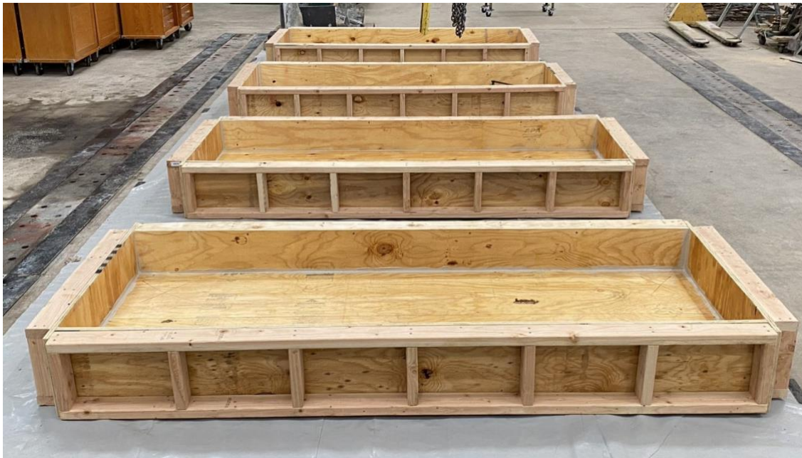
Figure 3-5: Formwork for four slabs
