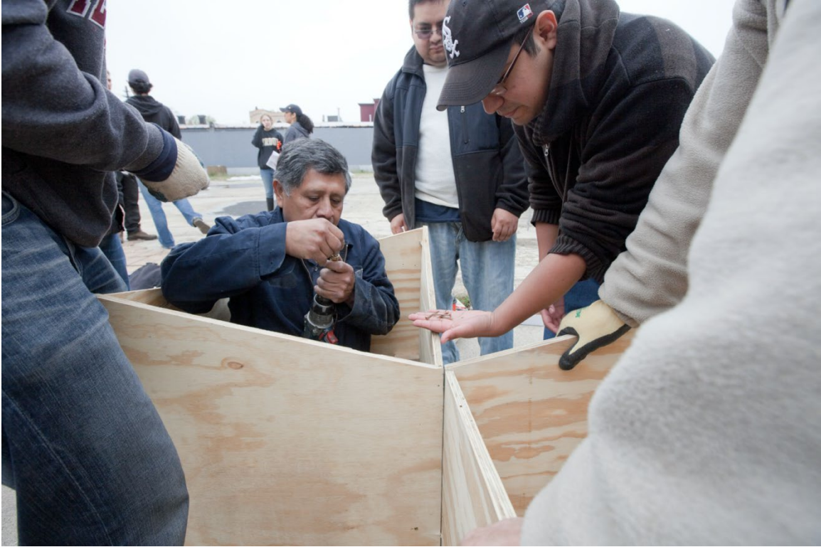
Figure 2: Assembly of MAS Studio's Cut. Join. Play. in Little Village, Chicago (Photograph by David Schalliol)
