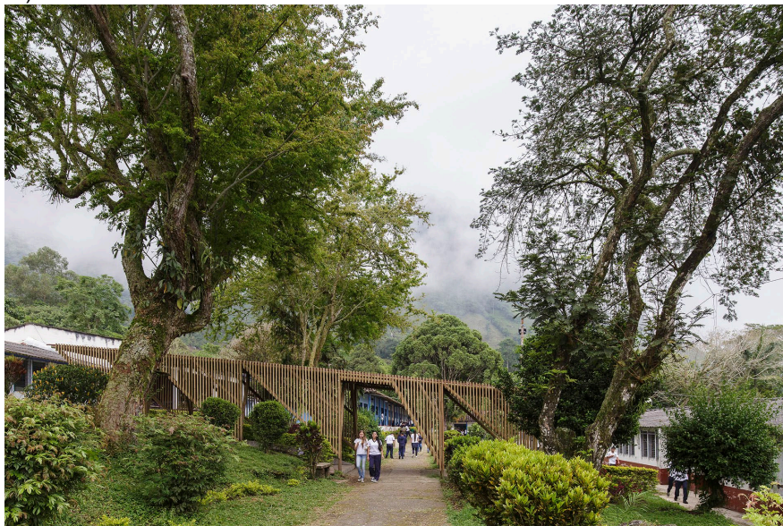
Figure 10: Covered walkway connecting two school buildings in Tâmesis (Alejandro Arango)
