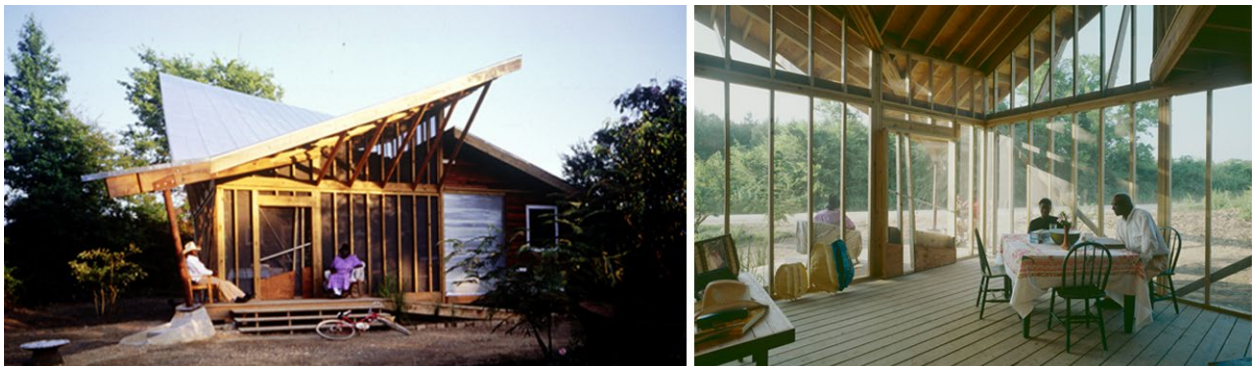
Figure 1: The Harris "Butterfly" House features a large roof that collects rainwater and a sizable porch for outdoor living. (Timothy Hursley)
