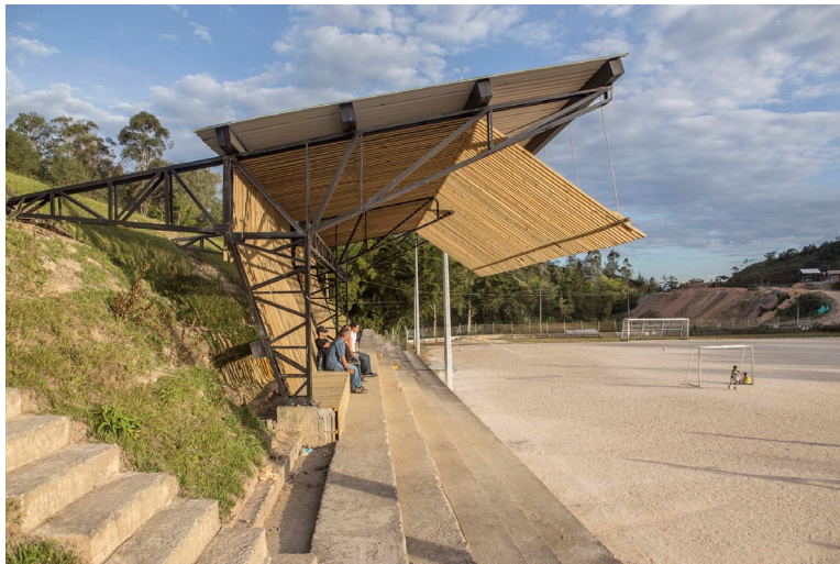
Figure 5: Sunscreen for the grandstand of a soccer field in San Vicente (Alejandro Arango)
