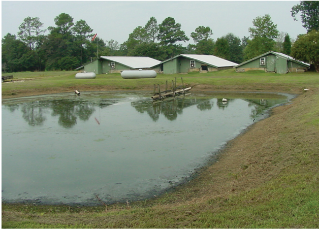
Figure 5. Alligator wastewater storage pond.
