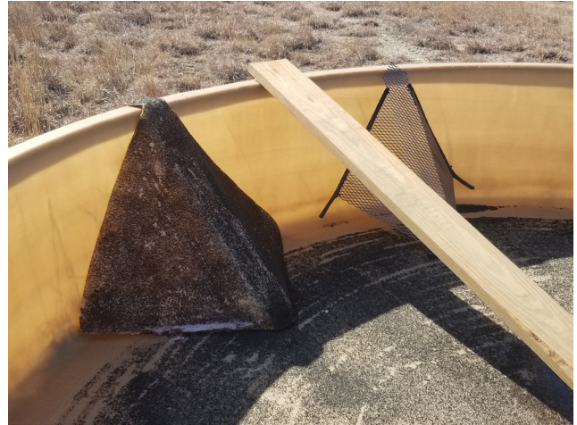
Various escape ramp designs exist. Whatever you use, make sure it is securely fastened and is positioned so animals swimming around the rim will intercept it. For example, the wooden board pictured here is not positioned correctly, but the wire and plastic ramps are. (Photo Courtesy of Weston Storer)
