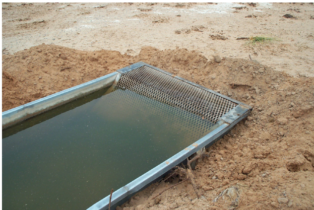
An example of a simple escape ramp that will prevent wildlife death and keep a clean water source available for livestock. (Photo courtesy of Roswell BLM)
