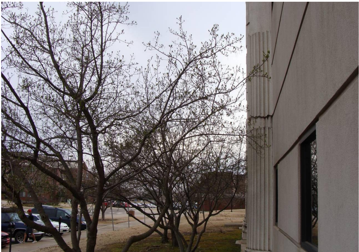
Figure 4: Trees touching the building
