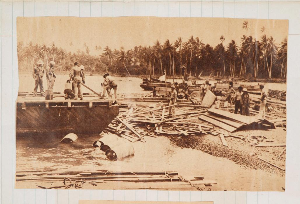
Ponton bridges of various types are included in the equipment of the Engineers. But sometimes boats to carry floating bridges are put together on the spot from whatever material may be available. Here barges are constructed on a beach in embattled New Guinea.
