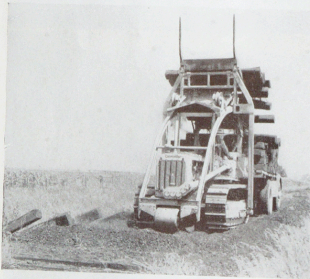
Top: "Big Boy" of the Union Pacific, with 16 drive wheels, pulls a mile of freight more than a mile a minute, "cruising" at 70. Center: Caterpillar Diesel uprooting and salvaging ties from a 60-mile abandoned railroad, loading ties into truck at rear. Below: An Elwell-Parker loading truck carries a pipe into a boxcar
