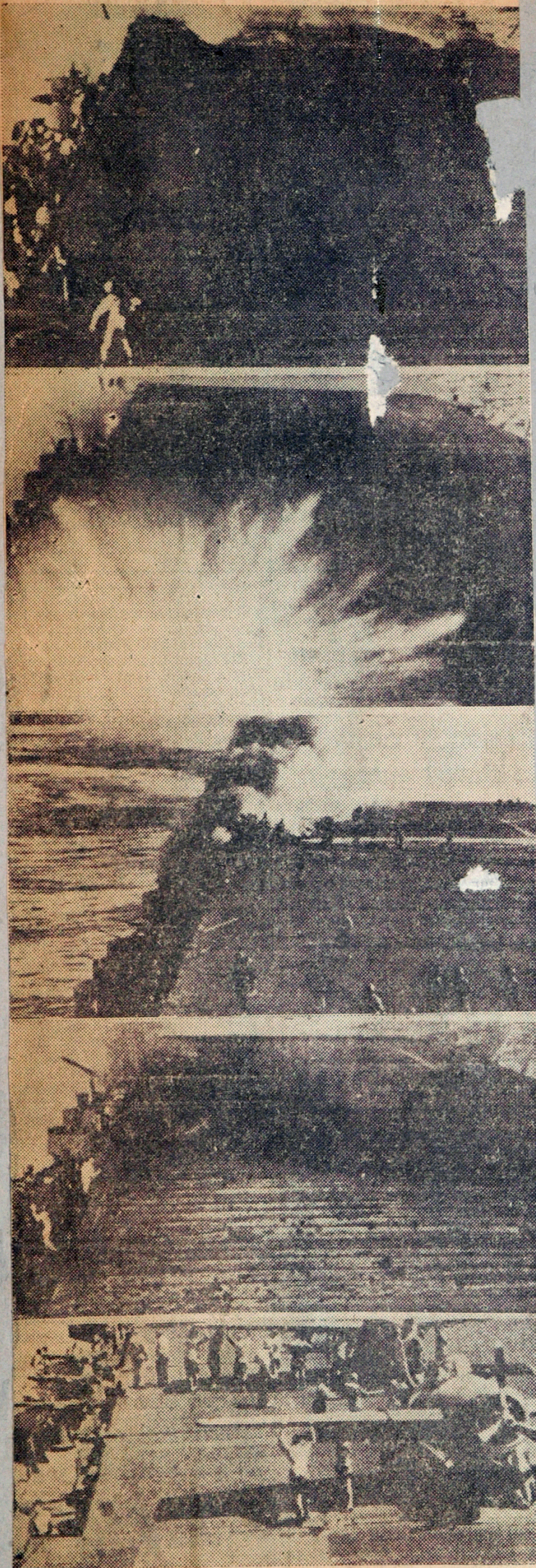
This series of action shots, official U. S. Navy photos taken aboard an American aircraft carrier in the Pacific war theater, shows quick action of the crew in fighting the fire that resulted from one hit and repairing another. In the top photo, the aft end of the runway is smouldering from a hit in that section. Next a fire-fighting crew attacks one menace while others rush to repair a crater left by the second bomb. Only a few moments later, as shown in the last photo, planes were on deck for action, the damage repaired.—(INS Soundphoto)
