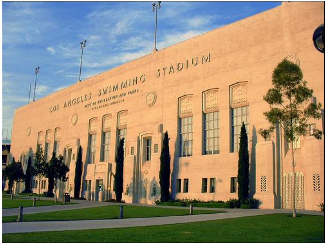
B-8: A modern view of the façade outside the Los Angeles Swimming Stadium. ( Photo from www.expositionpark.org ).
