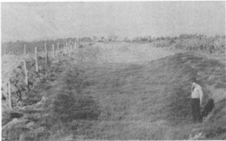
Fig. 10. Sodded outlet for outlet ditch.
