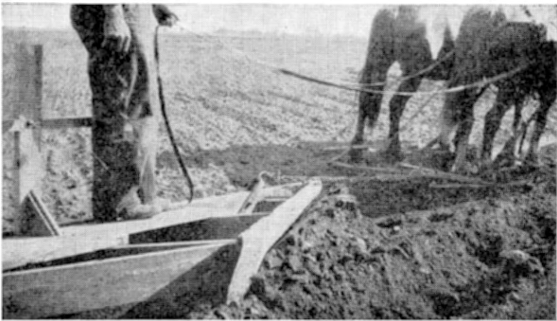
Fig. 7. —The terracer moving dirt. Notice the dirt rolling forward.
