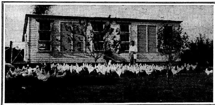
The extension poultry house improvement program is resulting in healthier chickens and better returns. Four hundred sixty-one new houses were constructed under extension agents supervision in 1932.
