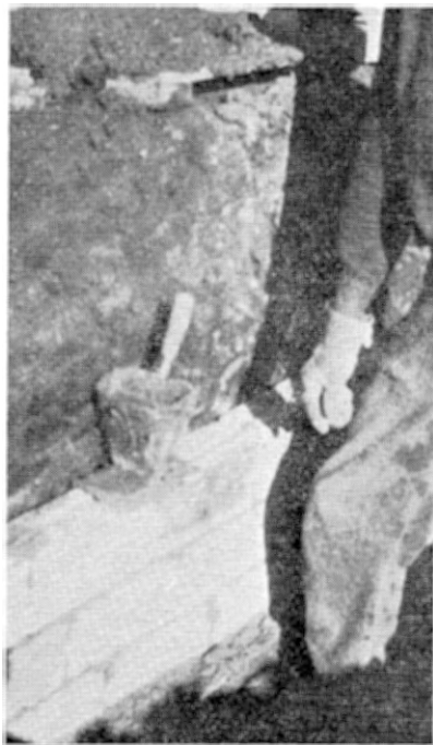
Fig. 3.—Shows the mortar being put in the vertical joints with the aid of a small mule.
