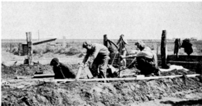
The drouth of 1934 stimulated the making and laying of homemade sub-surface garden irrigation tile, a project in Extension agricultural engineering.
