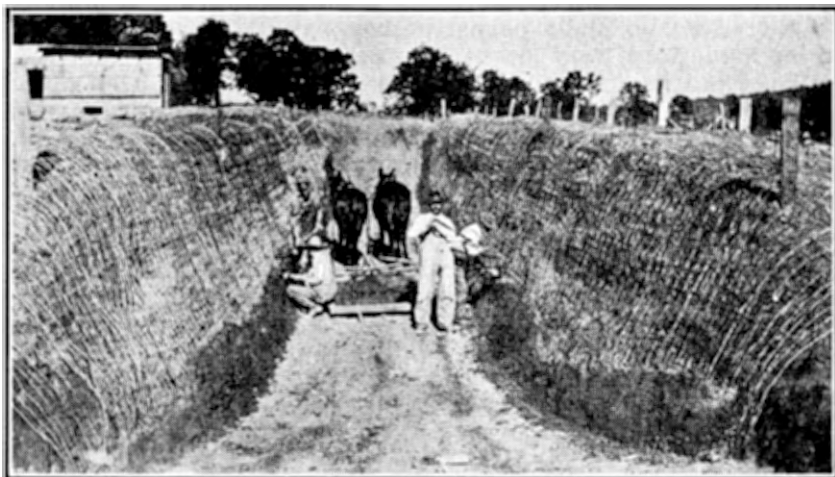
Building a Trench Silo
