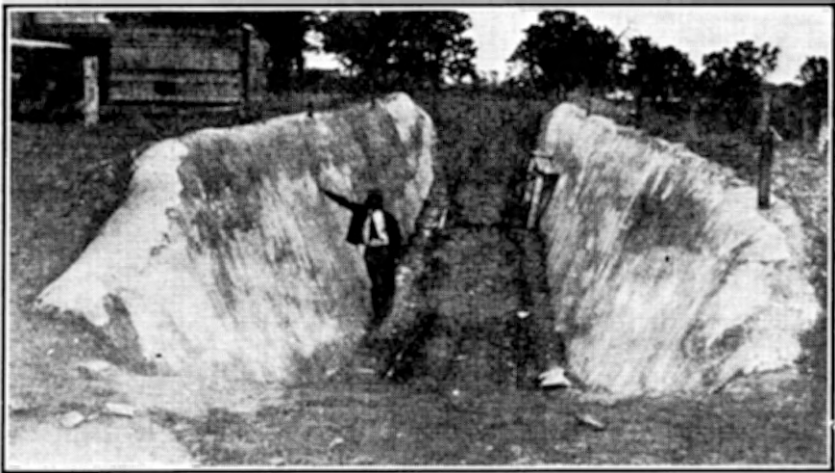
Fig. 6. —This is the finished concrete-wall trench silo.
