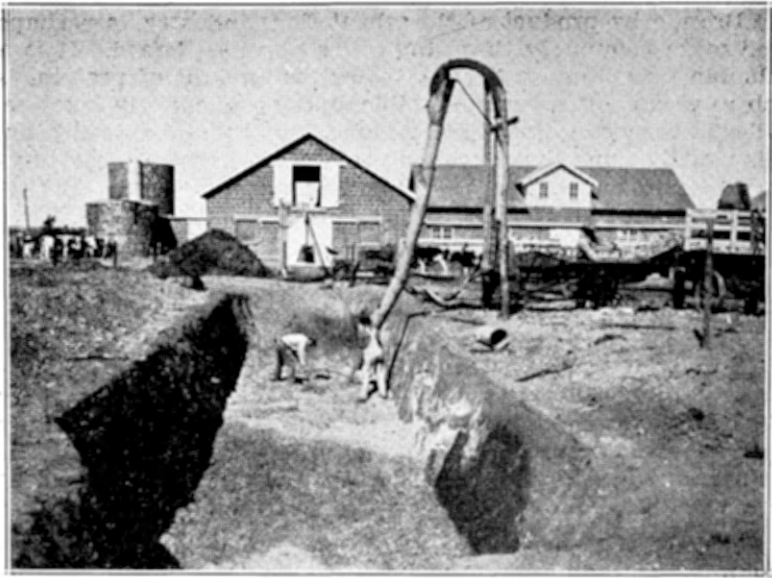
Fig. 3.—The trench silo provides an economical means of preserving a succulent dairy feed for winter or drouth periods when it cannot be obtained from other sources.
